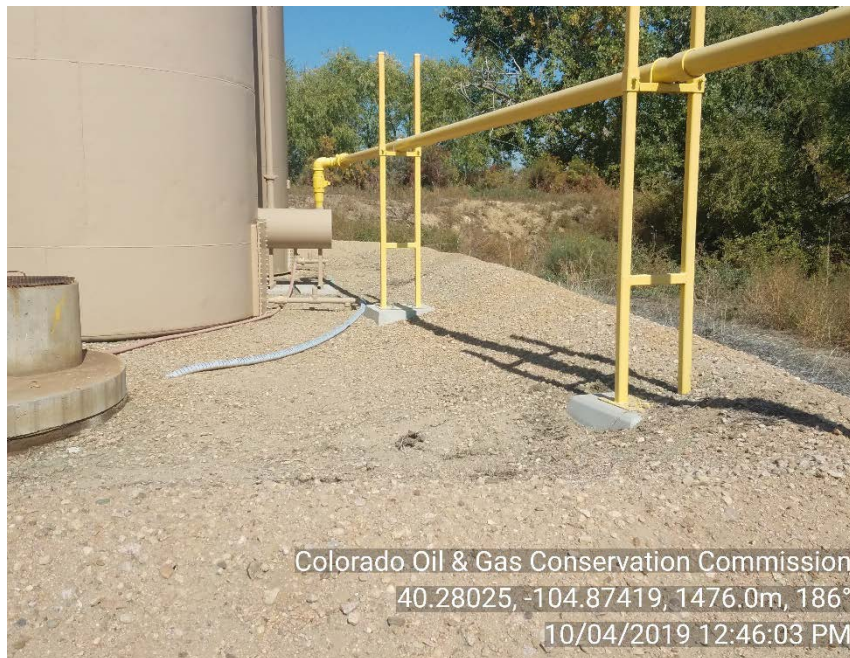
Crude oil tank berm
