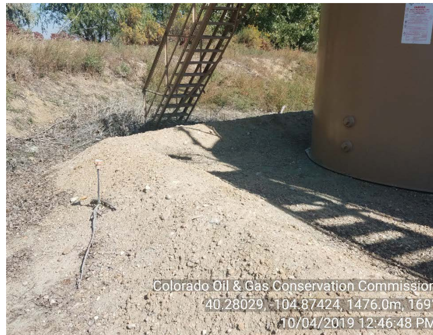
Crude oil tank berm
