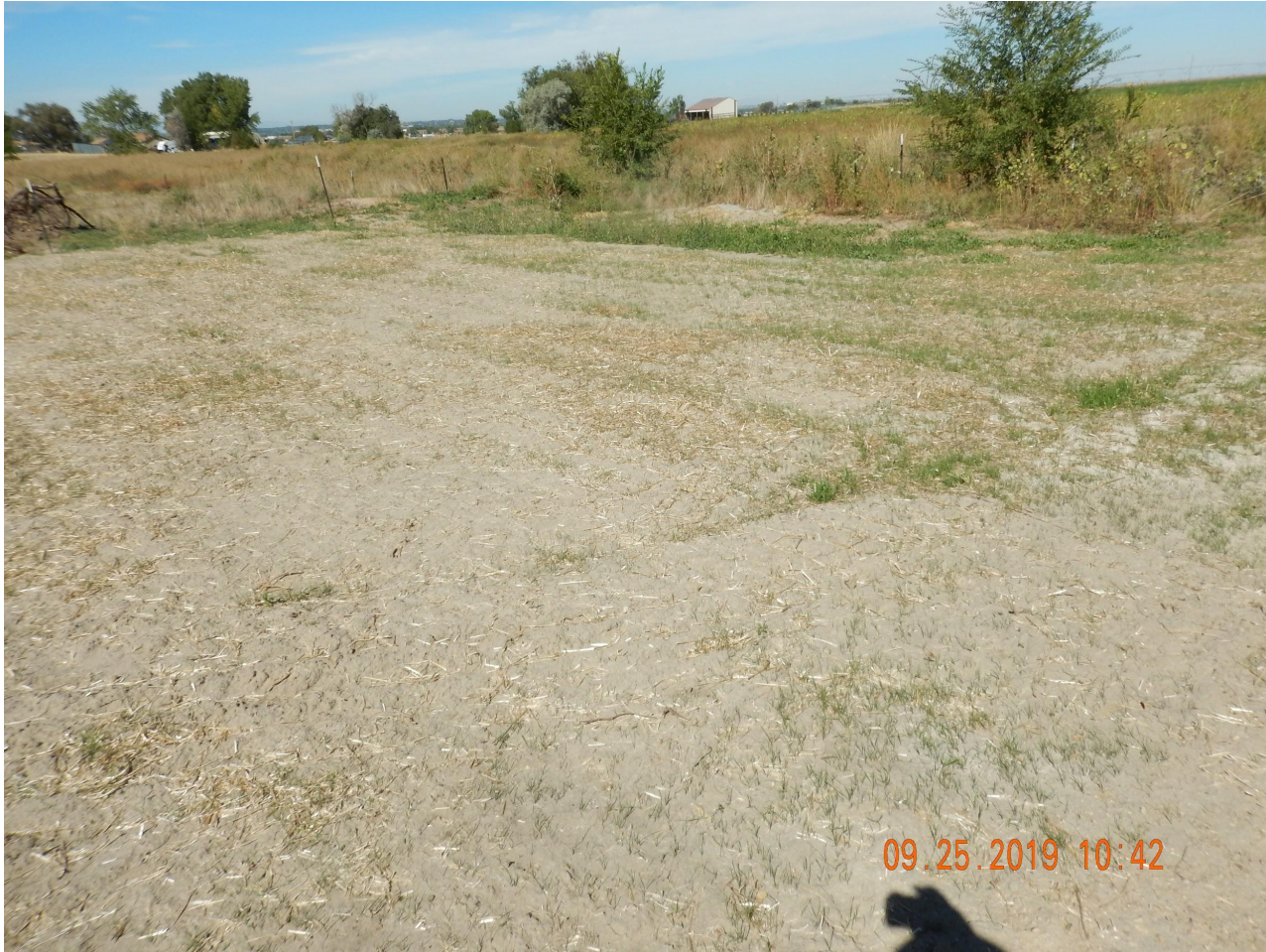
Photo 1. Photo taken from the southern tank battery, facing Northwest. Photo illustrates the Operator has performed Final Reclamation activities with the evidence of drill rows, straw mulch and germination.
