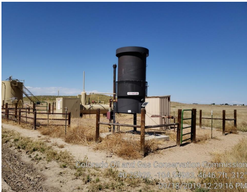
Photo #1 Separator, ECD, Meter Run & Weeds on 9/18/19
