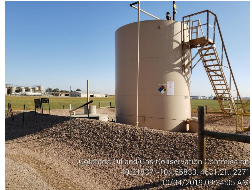
Photo #4 Tank Battery
