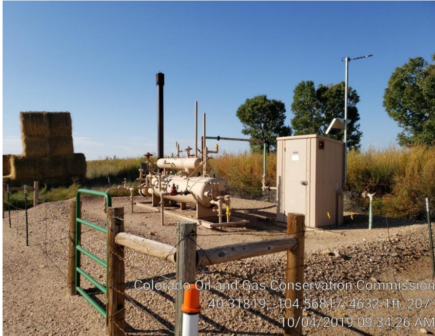
Photo #5 Separator & Meter Run
