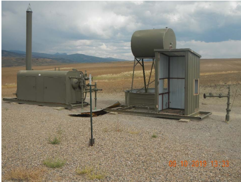
Photo 2. Meter run that has become debris. Unmarked riser on right side of meter run.
