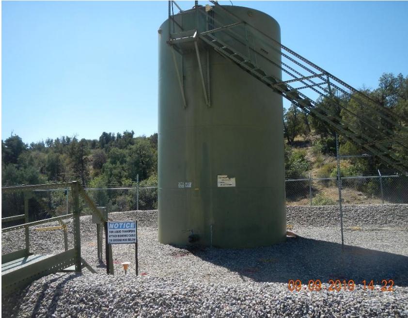
Heated AST does not have signage required by Rule 210.d.
