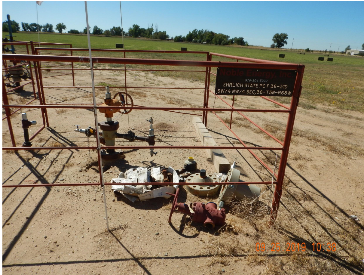
Photo 7. Photo taken from the nearby well (API#123-32549), facing South. Photo illustrates unused equipment that shall be removed per Rule 603.f.
