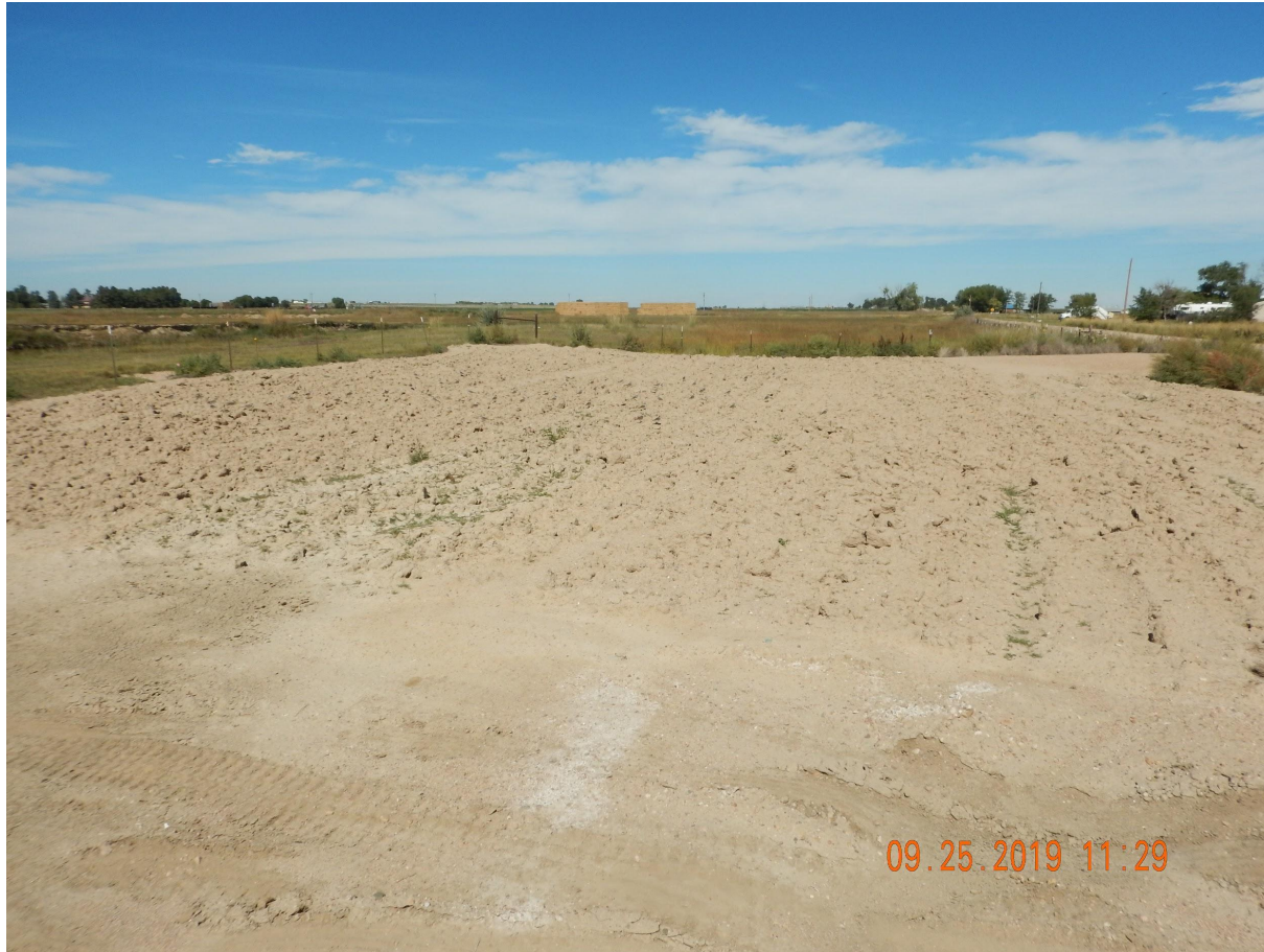
Photo 3. Photo taken from the southern portion of the northern tank battery, facing North. Photo illustrates the Operator has started to perform Final Reclamation activities as road base material has been removed. Appears compaction alleviation has been performed. It is unclear whether or not compaction alleviation has been cross-rippled per Rule 1003.c.
