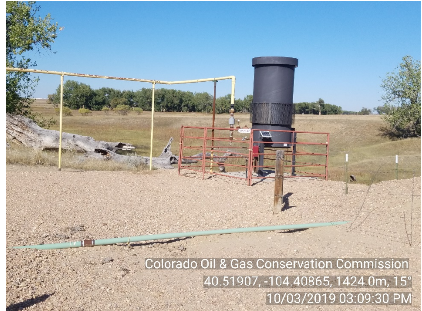
Photo #6 Brown 22-2 Battery NE Corner – Stormwater erosion NOW Appears mitigated
