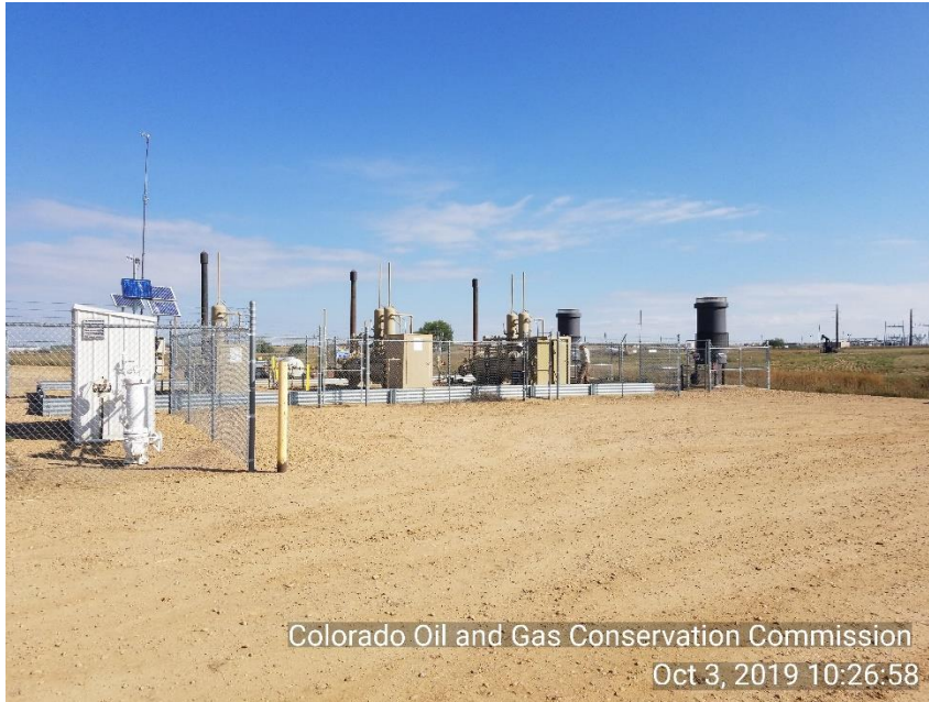
Photo 3 Sep/meter house and ECD's, crew onsite cleaning separator to be removed.
