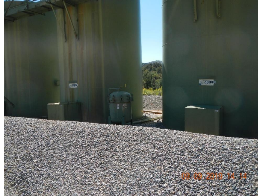
ASTs were not labeled with NFPA placards at the time of this inspection.
