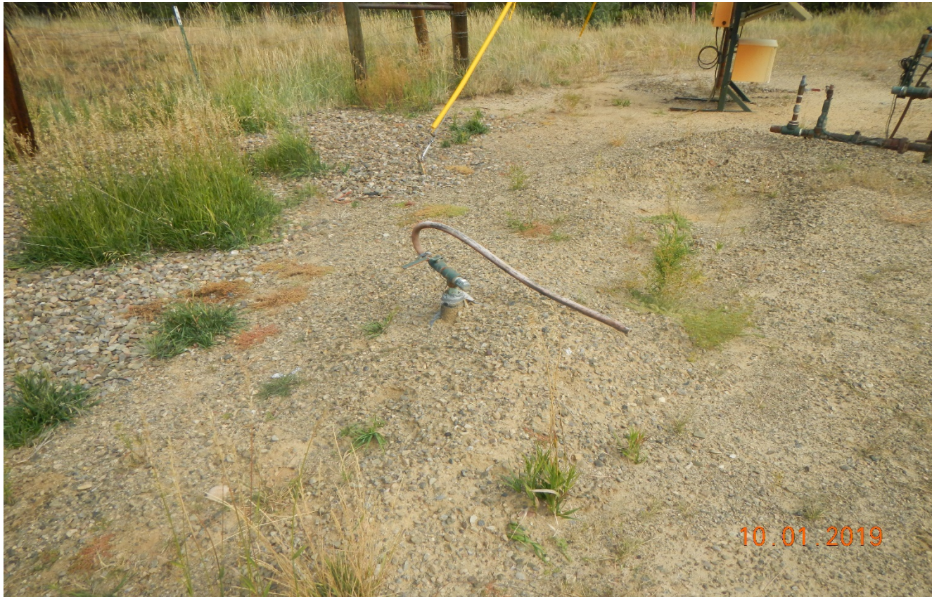
Photo 3. Unknown riser line with no LOTO.
