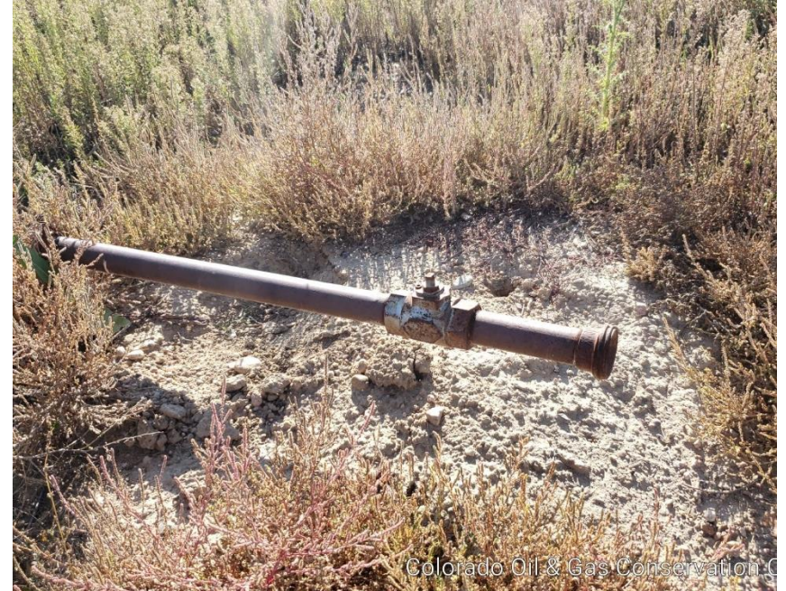
Photo #2 Unused unmarked flow line NO LOTO
