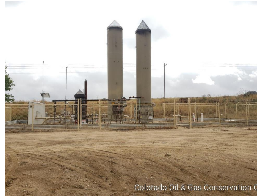
Photo #2 Meter house, ECDs and separator
