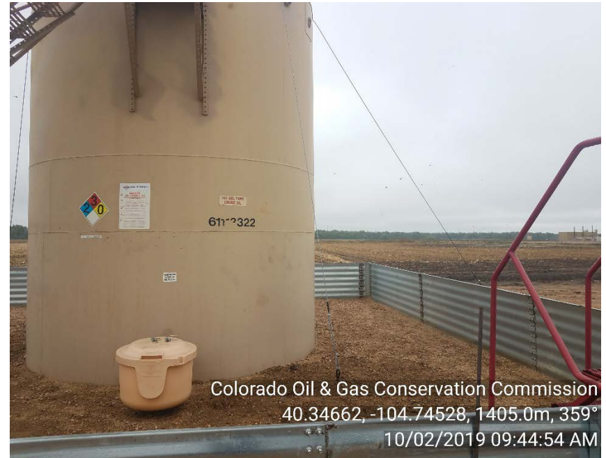
Crude oil tank anchoring
