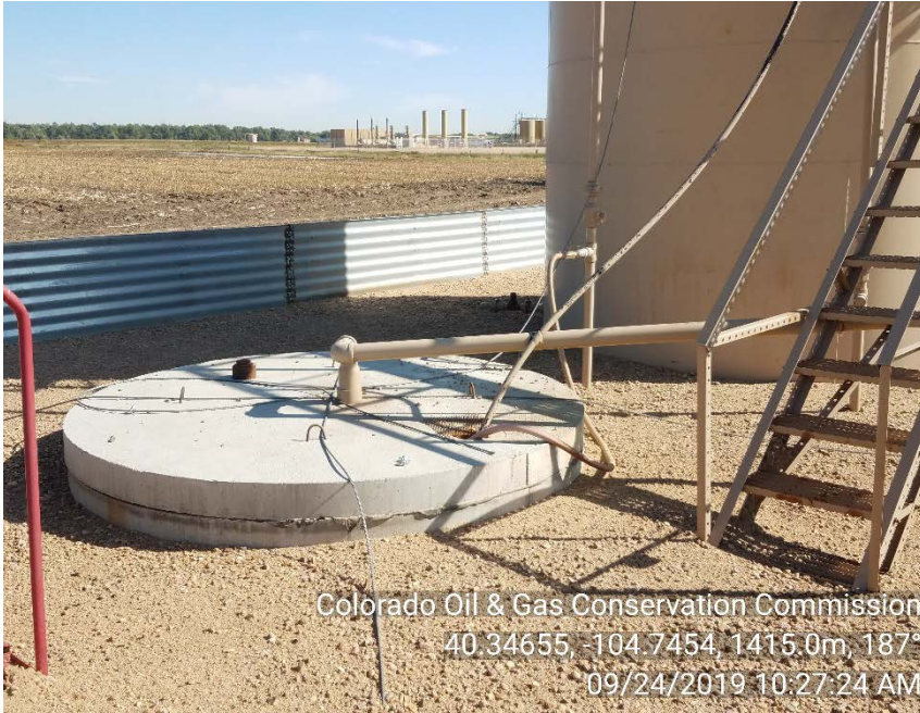
Crude oil tank anchoring on 9/24/19
