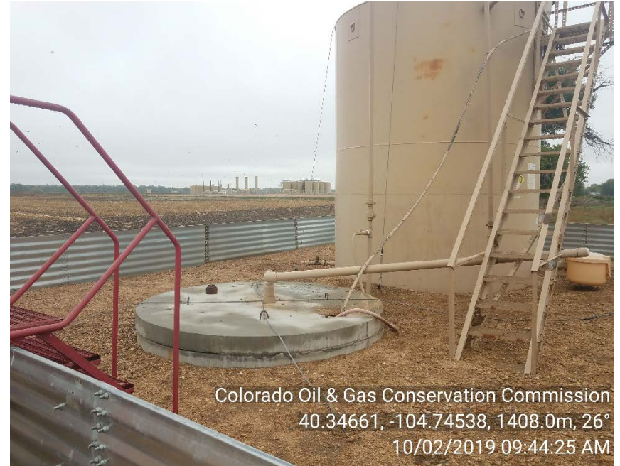
Crude oil tank anchoring on 10/2/19
