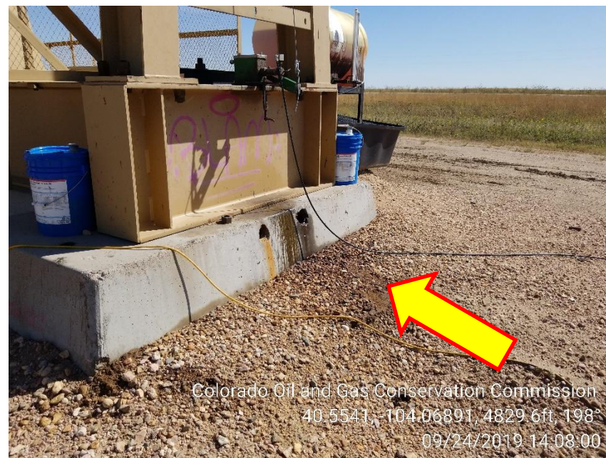
Photo 6 – Stained Soil at the front of the Pumping Unit
