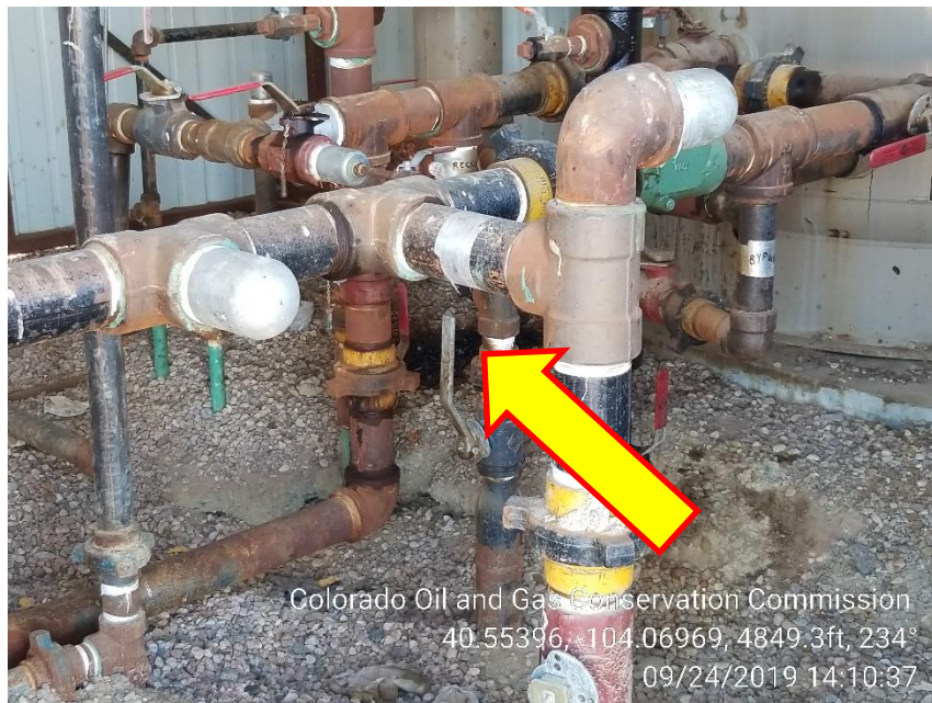
Photo 11 – Stained Soil at dumps inside the Treater Shed
