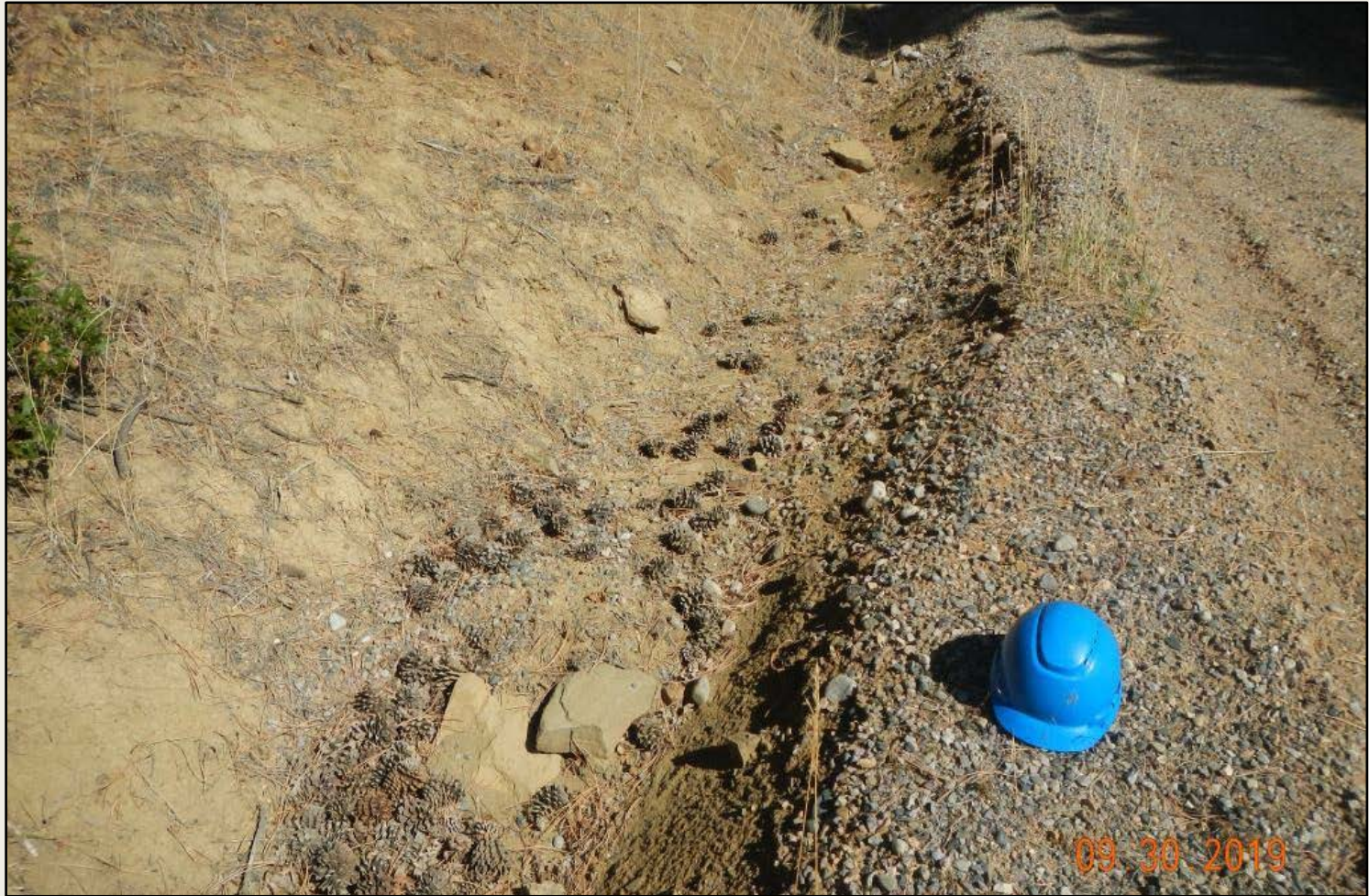
Photo 2. View of erosional downcutting (approx. 2 feet wide and deep) occurring along the access road where stormwater controls are needed.
