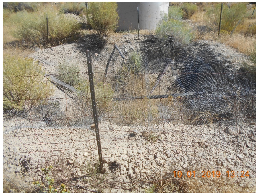
Pit with fence and netting
