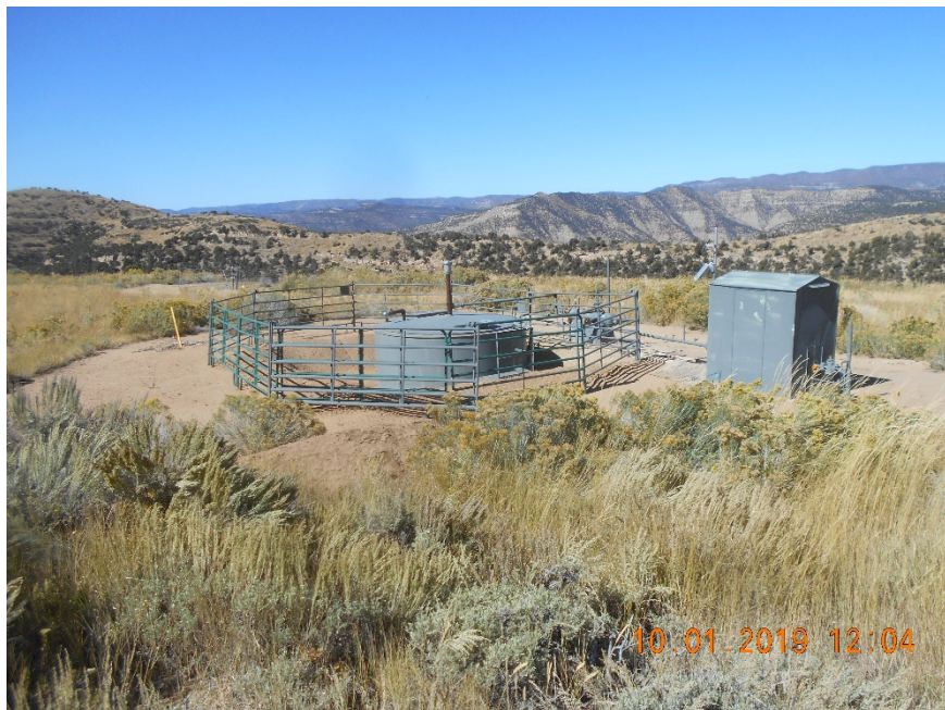
Location overview looking SW.
