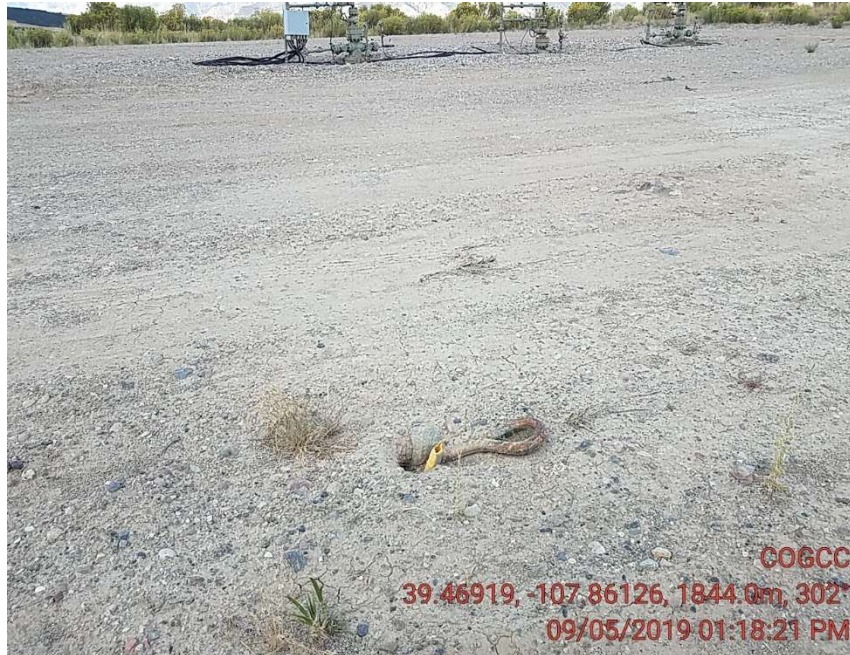
Unmarked dead man from previous inspection
