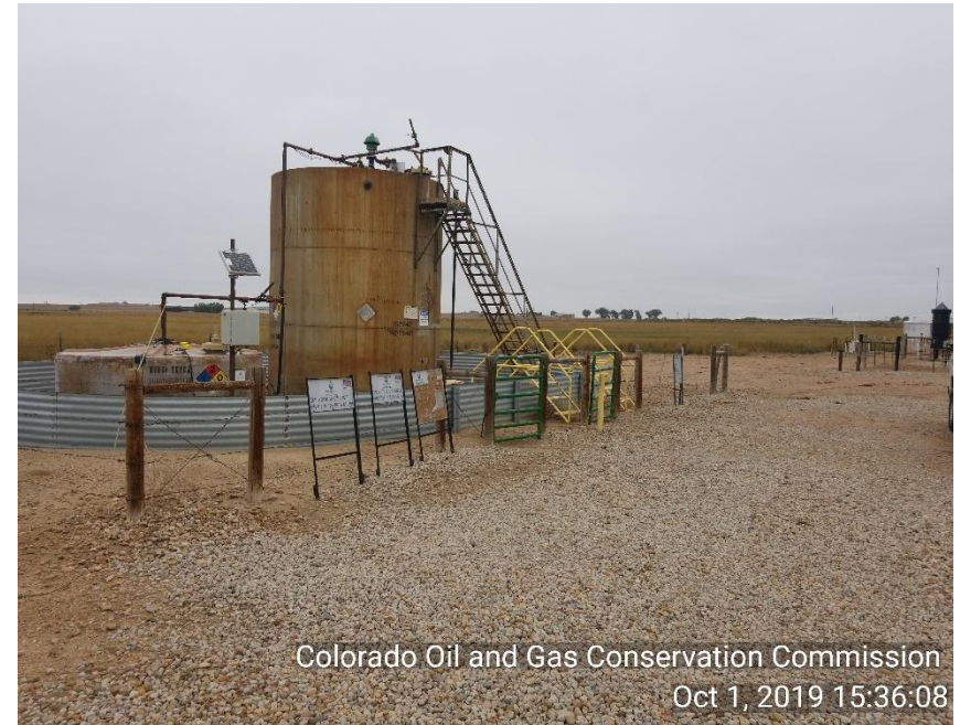
Photo 4 TNK BTRY. Crude oil tank visible from public road paint is covered by what appears to be rust
