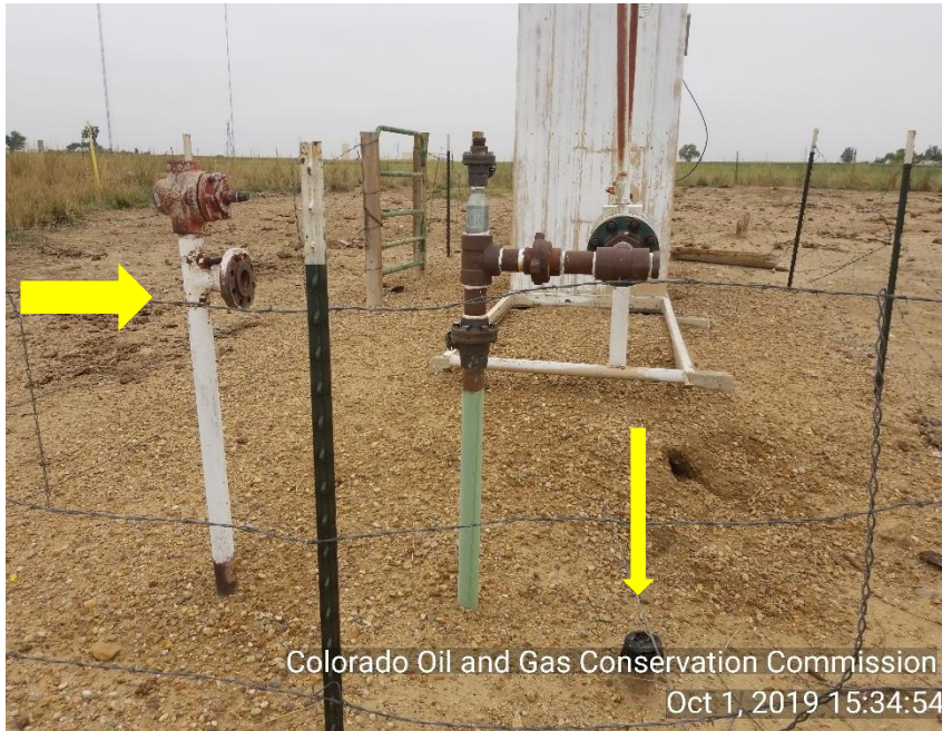
Photo 3 Unused equipment: unmarked not LOTO risers
