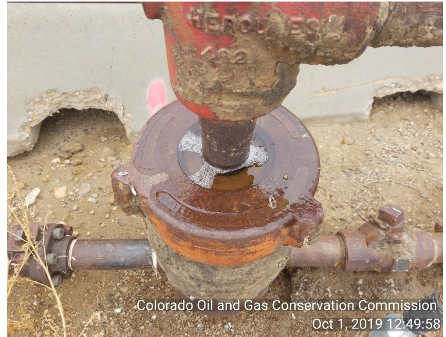
Photo 4 VENTING: bubbles show what appears to be well head leaking at the tubing.
