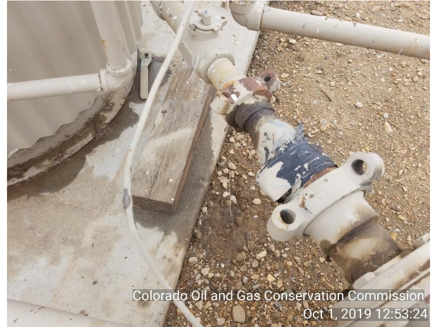
Photo 12 Stained soil and mechanical issues on Vertical heated separator.
