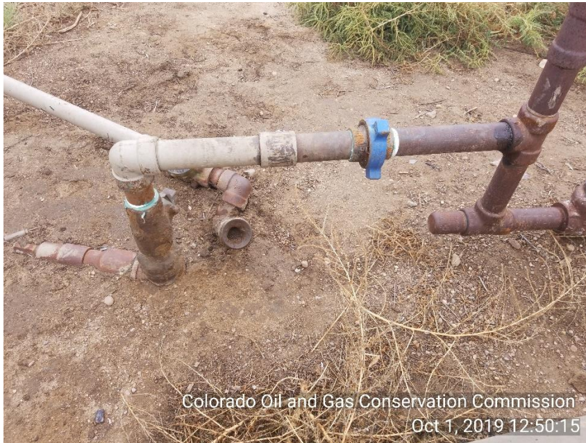
Photo 5 unused equipment: Unmarked not LOTO riser on flow line.
