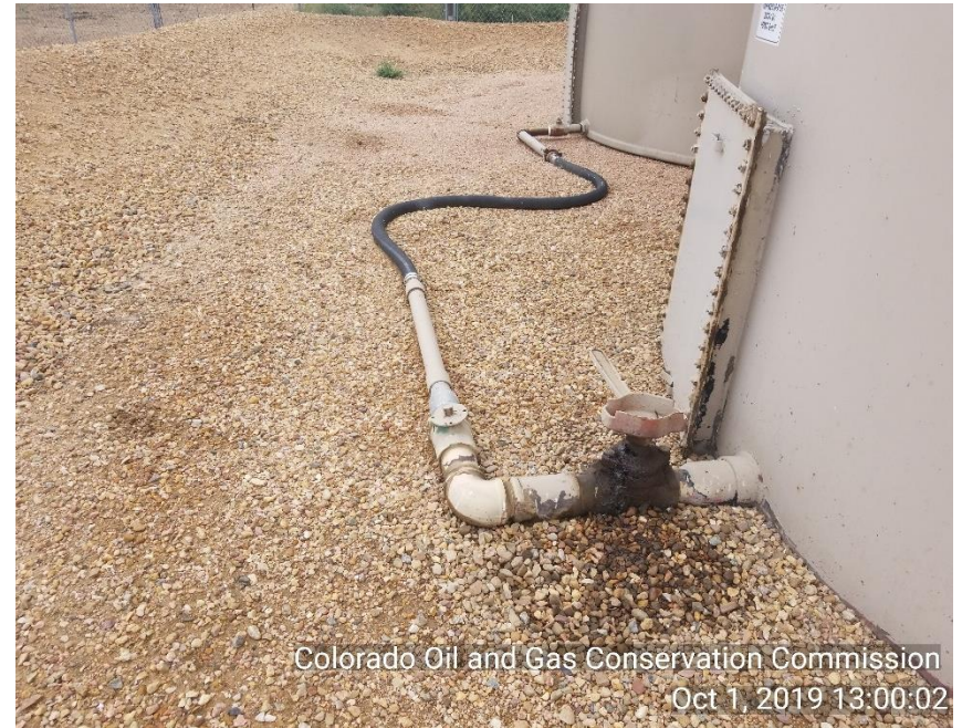
Photo 10 stained soil around crude oil tank load line.
