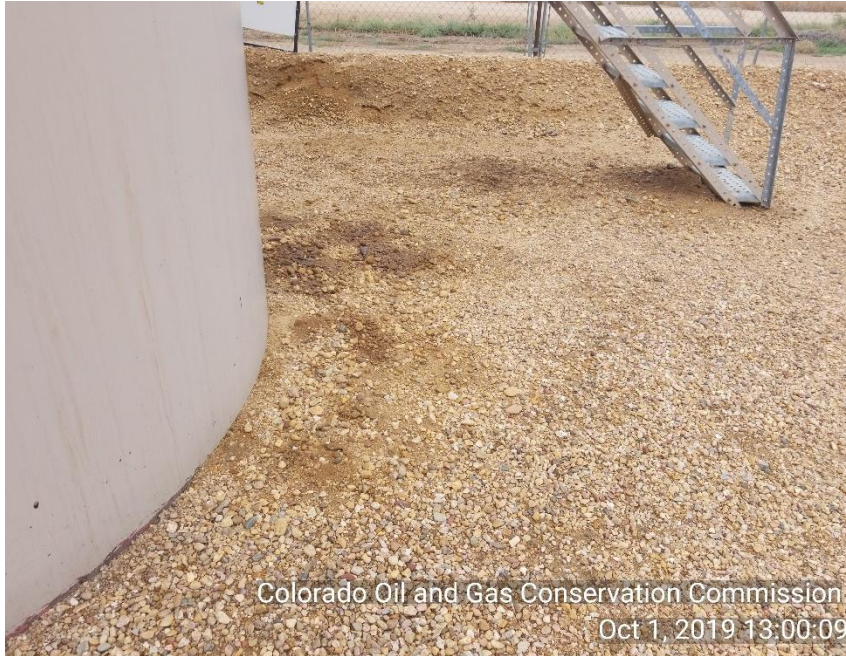
Photo 11 stained soil around crude oil tank
