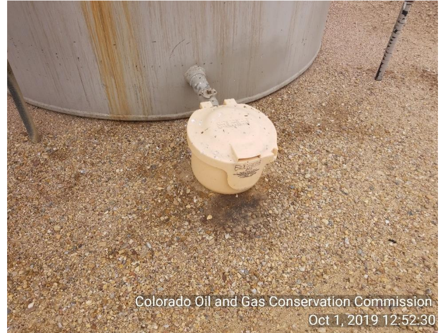
Photo 8 Stained soil under Produced water load line.
