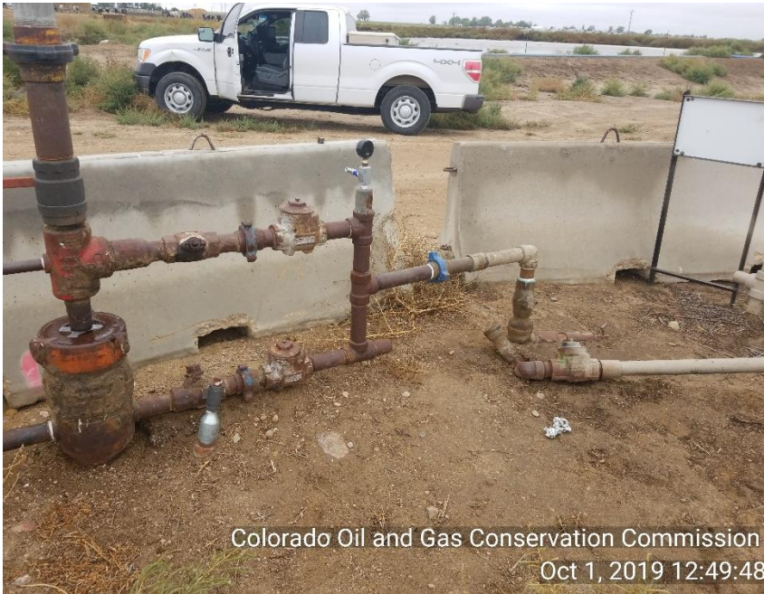
Photo 3 appears KPK has hooked up production lines from well head to vertical separator since last inspection and opened flow line valves.
