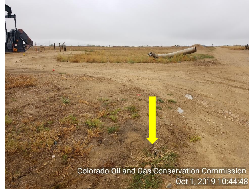
Photo 10 Storm water BMP: Culvert outlet and drainage ditch not maintained. Top of culvert exposed not proper cover at entrance to well site.
