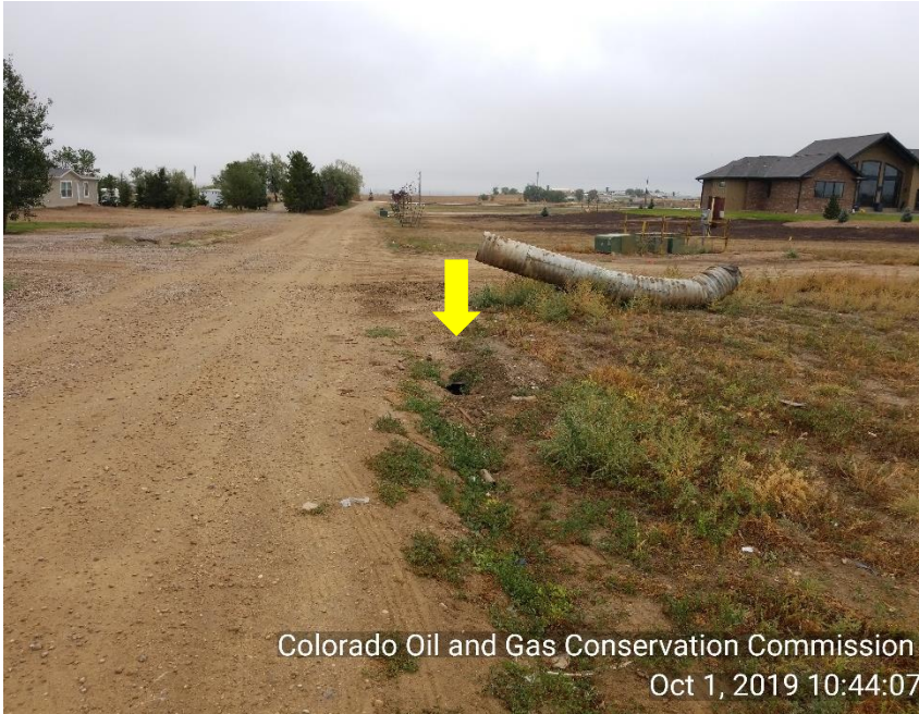
Photo 9 Storm water BMP: Partial culvert removed and drainage ditch and to opening of culvert not maintained at entrance to well site.
