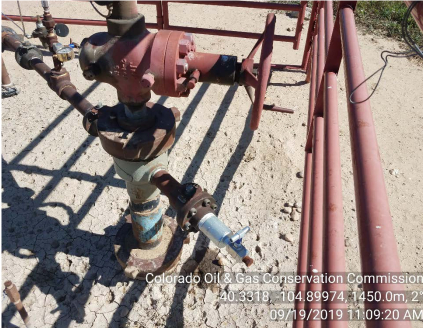
Master valve and stained soil on 9/19/19
