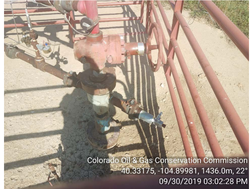
Master valve and stained soil on 9/30/19
