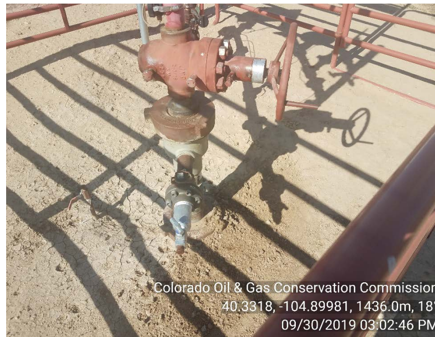
Master valve and stained soil on 9/30/19
