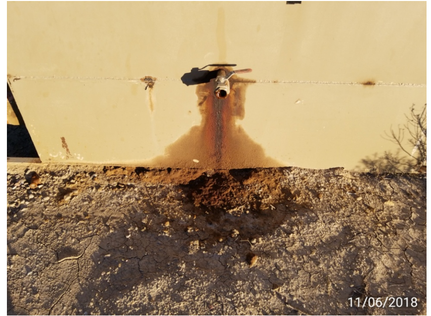
Photo 7. Separator leak – 11/06/2018
