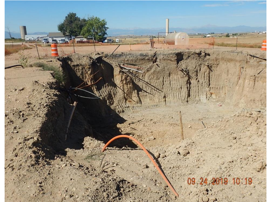
Cut ends of flowlines exposed in excavation (view to west).
