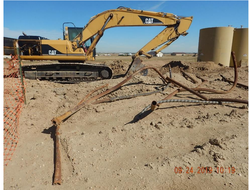
Flowline segments cut out/ removed from excavation.
