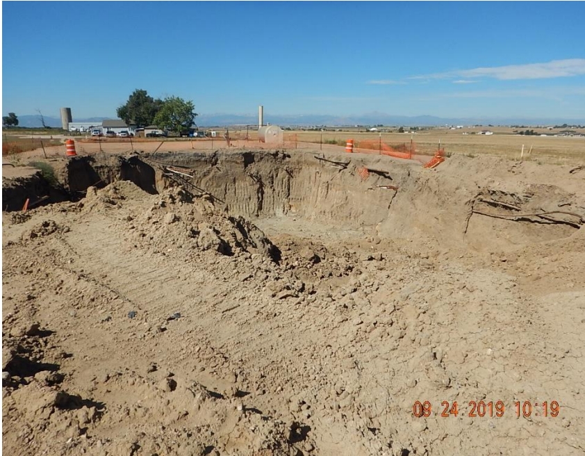
View of excavation (flowlines exposed in walls/ view west).
