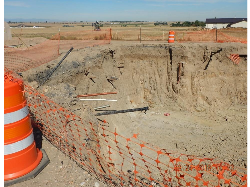
View of excavation (flowlines exposed) looking NW.
