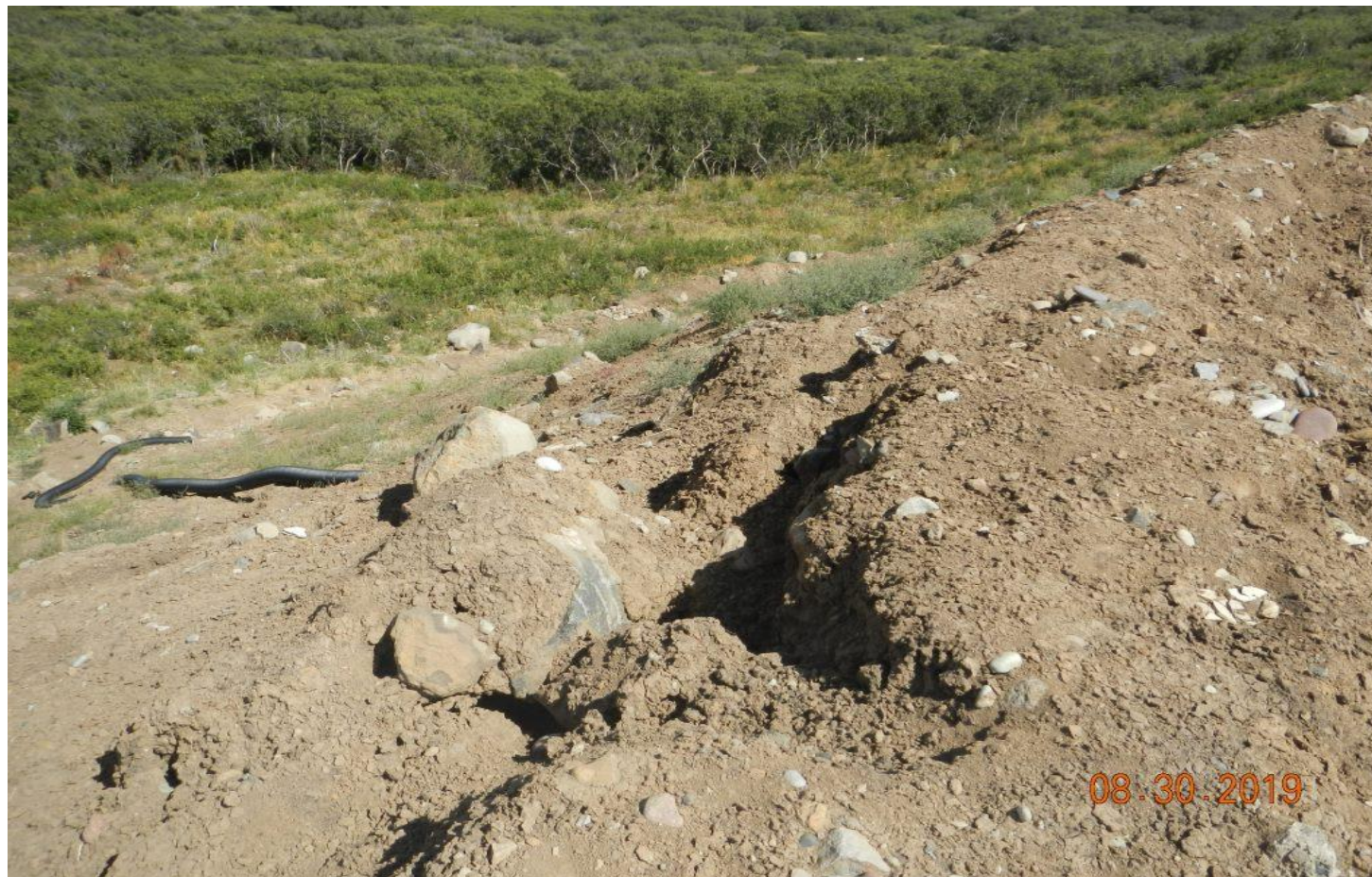
Photo#6: Fill slopes are not stable.
