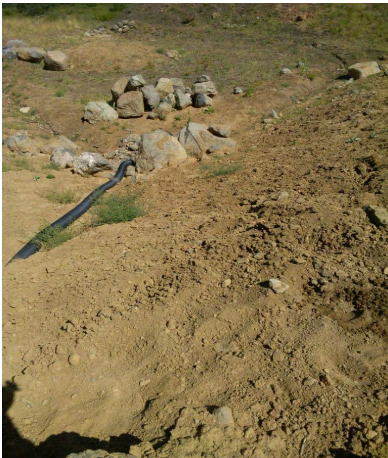
Photo#7: Fill slopes are not stable
