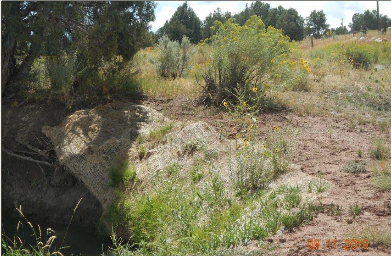
Photo 14. View of straw blanket on bank at location detailed in Photo 13. Vegetation appears to be progressing on this bank, through the blanket material.
