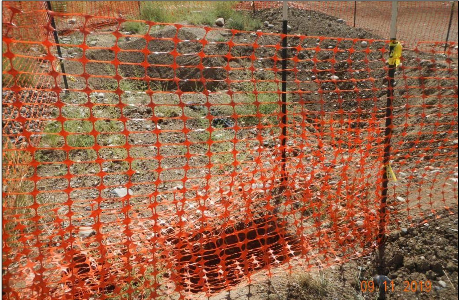
Photo 6. View of holes within the project area. Fencing is not sufficient to mitigate wildlife risk, and holes need to be filled.
