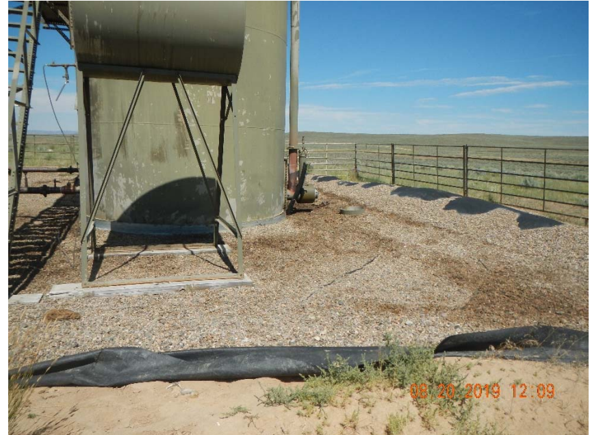
Photo 2. Non reportable spill – stained gravel in tank battery.
