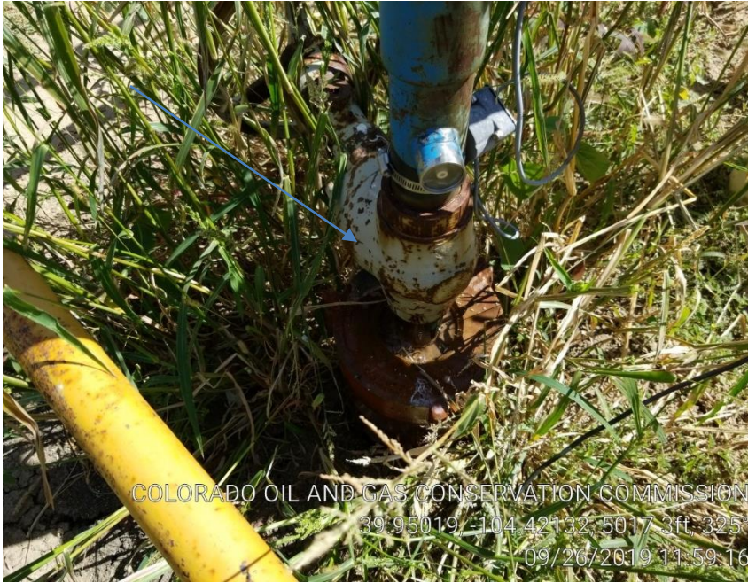
Pic 3 venting wellhead
