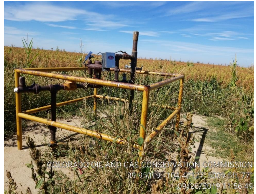
Pic 2 wellhead no sign
