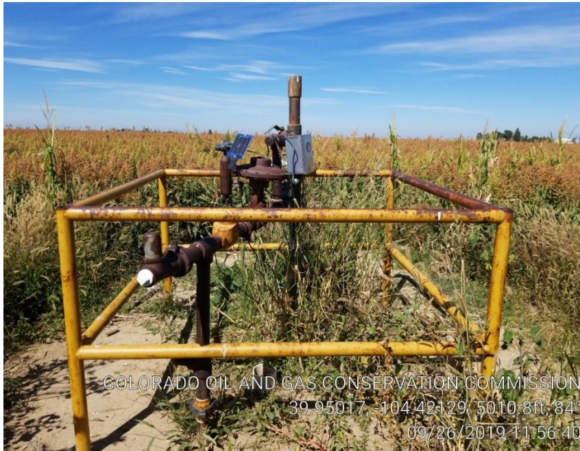
Pic 1 wellhead no sign
