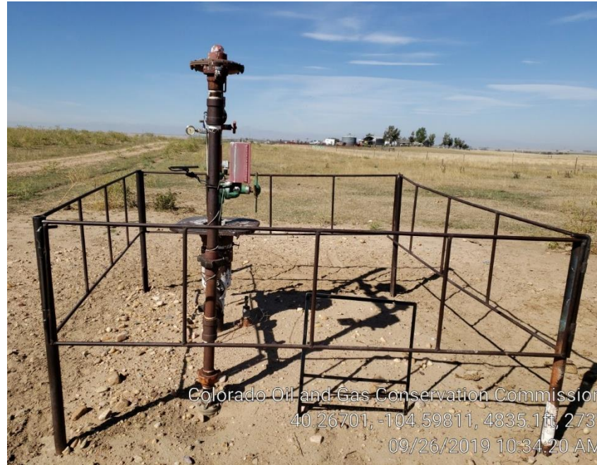
Photo # Wellhead & Missing sign
