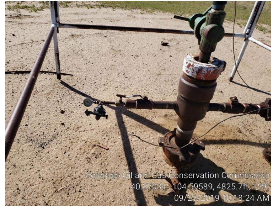
Photo #2 broken stainless line that runs motor valve.
