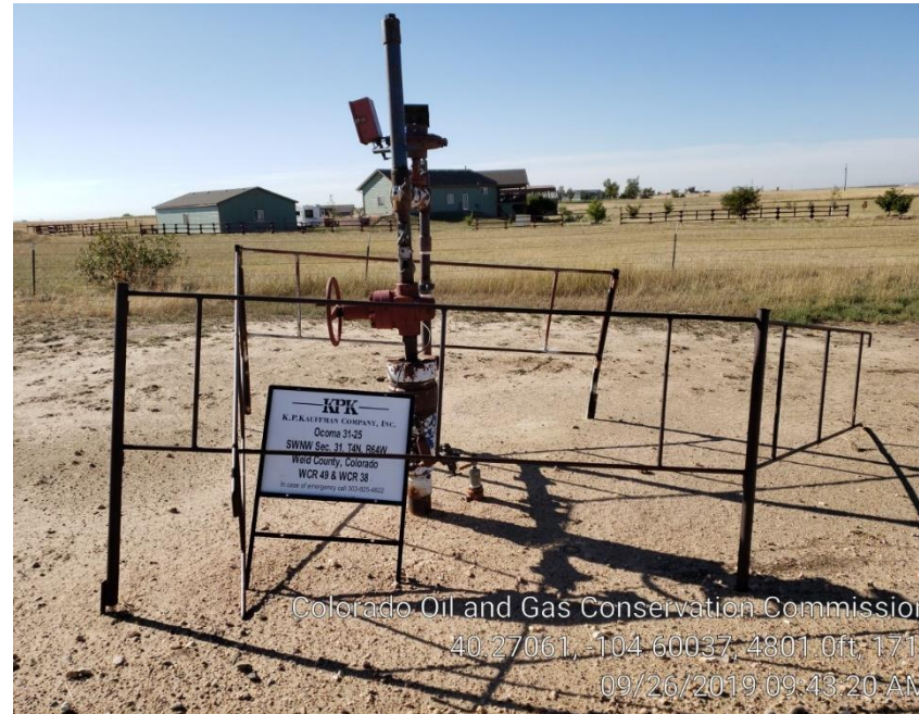
Photo #1 Wellhead, Sign, & tore down fence.
