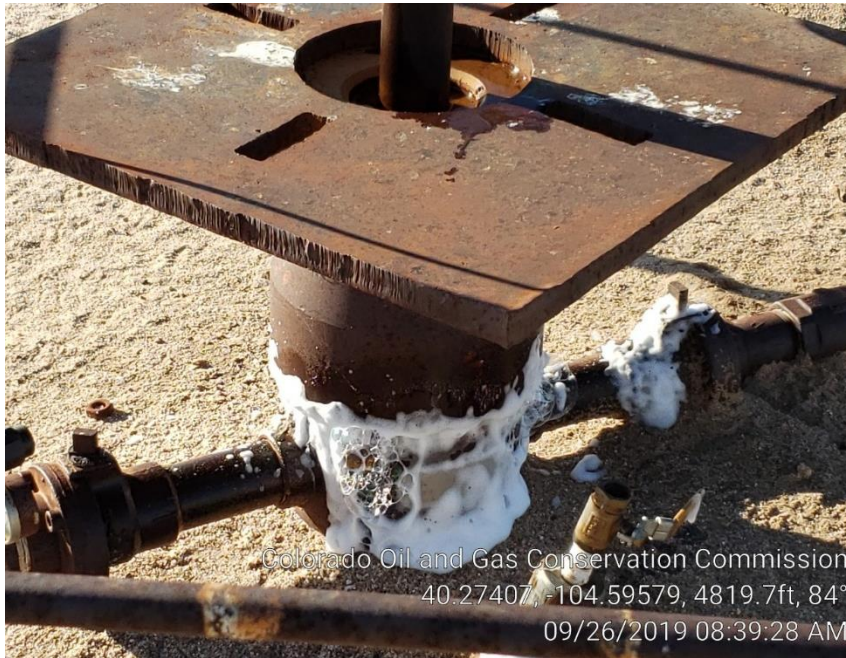
Photo #2 Active leak at the casing collar
