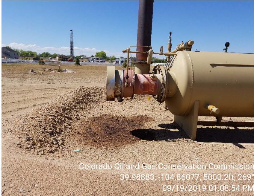
Photo 5 – Stained soil under fire tube
