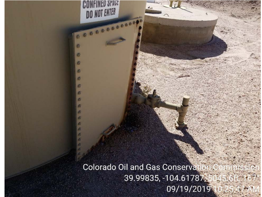
Photo 4 – Stained soil at crude oil tank access panel
