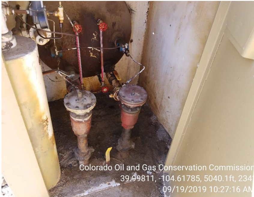
Photo 5 – Stained soil at separator
