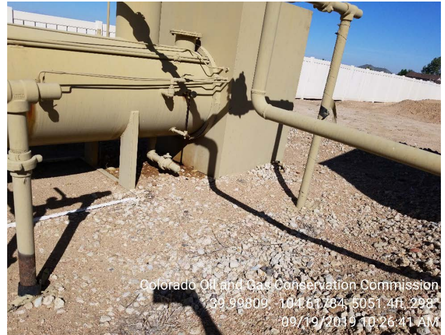
Photo 6 – Stained soil at separator
