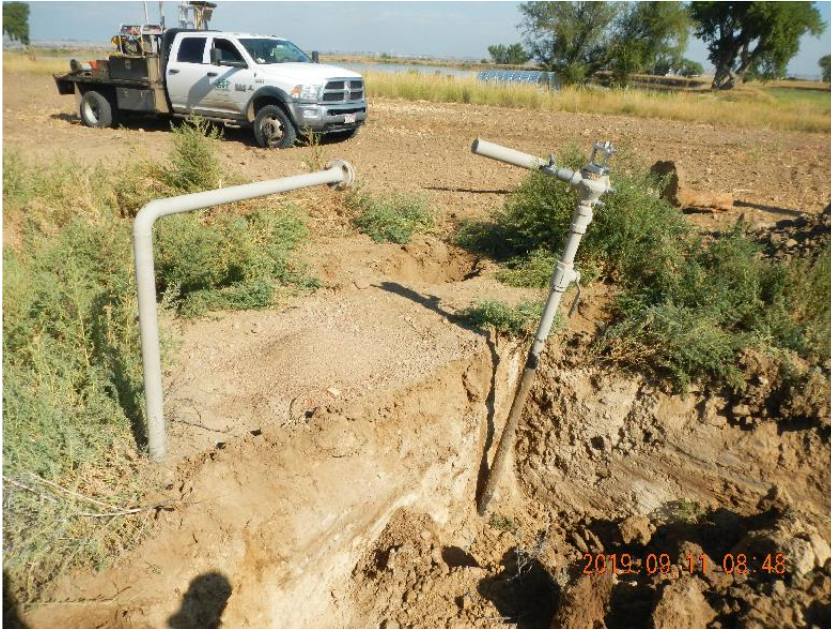
Photo 3: Risers with construction fencing removed and excavation started.
