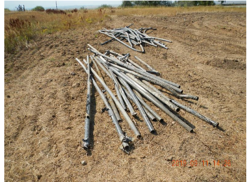
Photo 10: Removed flow line piled for haul off.
