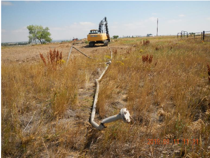
Photo 7: Removed riser and flow line.
