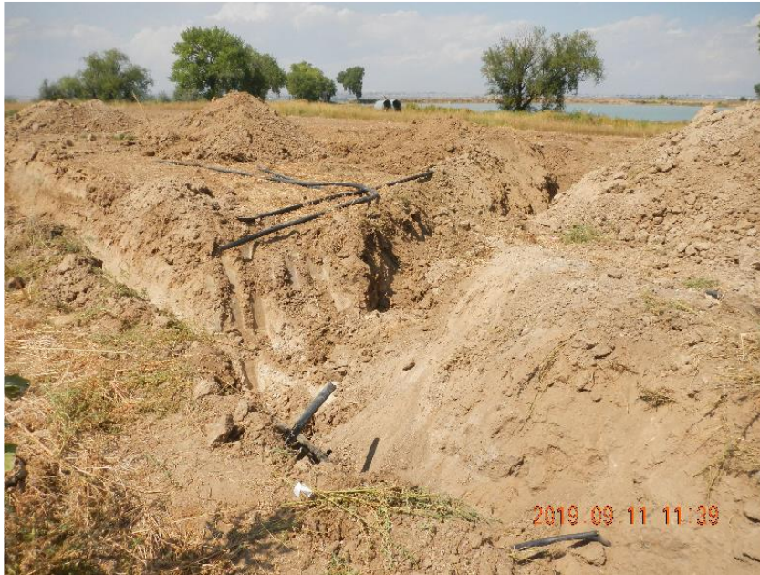
Photo 9: Excavation heading SE removing separator to tank flow line.
