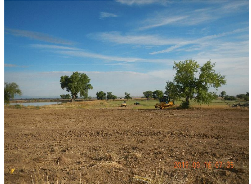
Photo 14: Site looking S after backfill and leveling.
