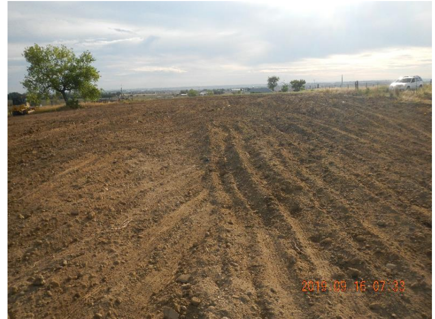
Photo 12: Site looking W after backfill and leveling.
