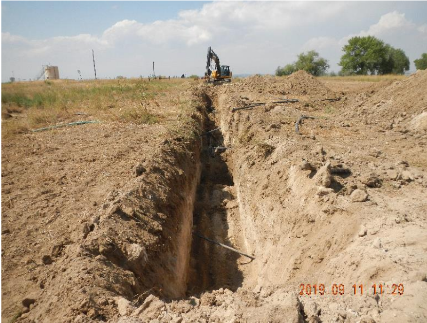
Photo 5: Long view of excavation trench looking E from old separator site.
