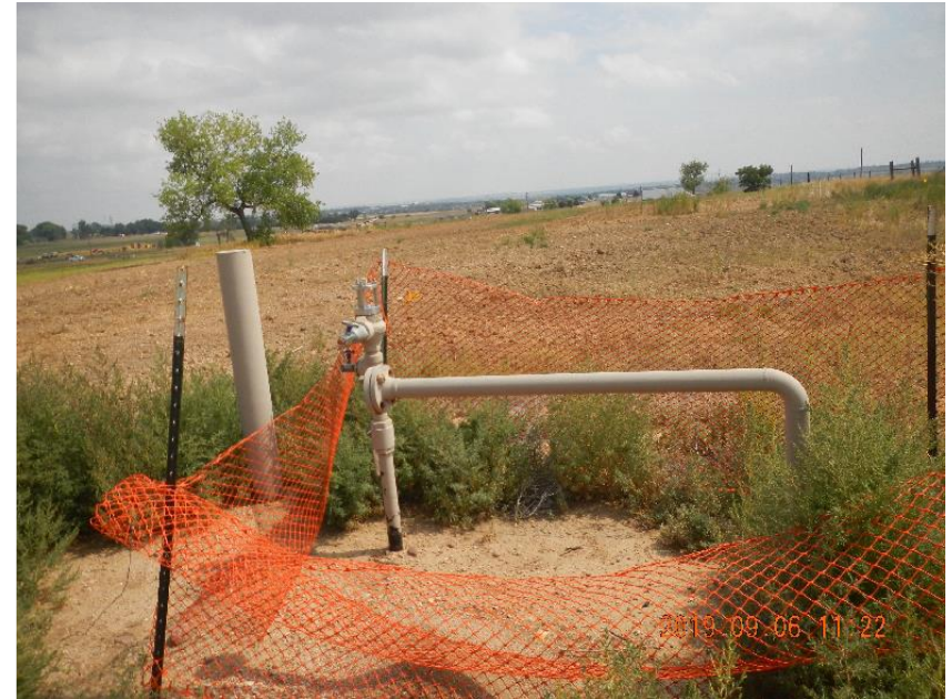
Photo 2: Close up view of risers to be removed.
