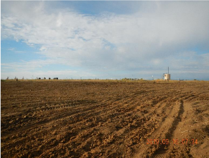
Photo 13: Site looking N after backfill and leveling.
