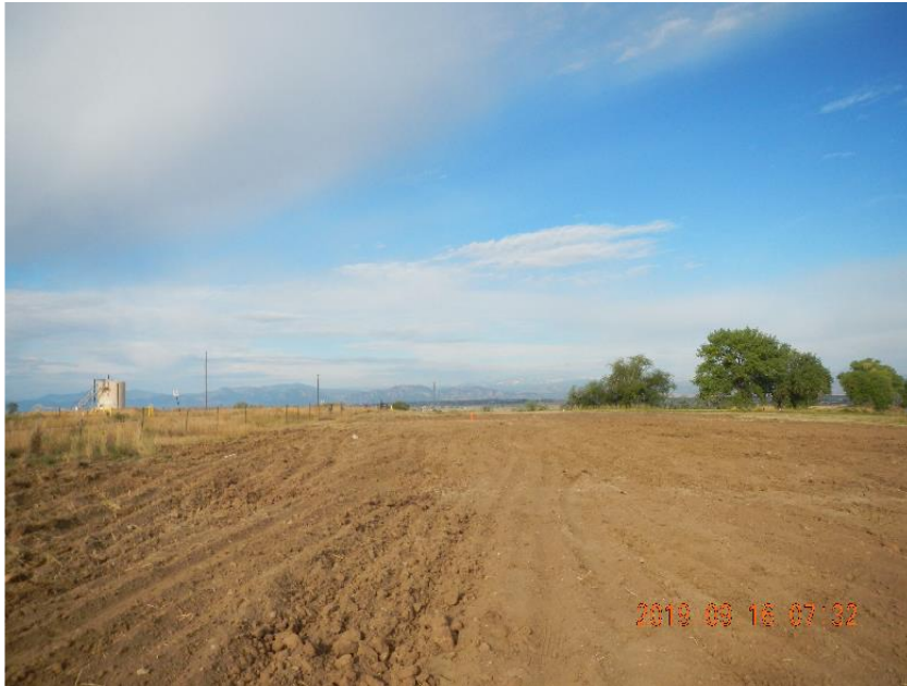
Photo 11: Site looking E after backfill and leveling.
