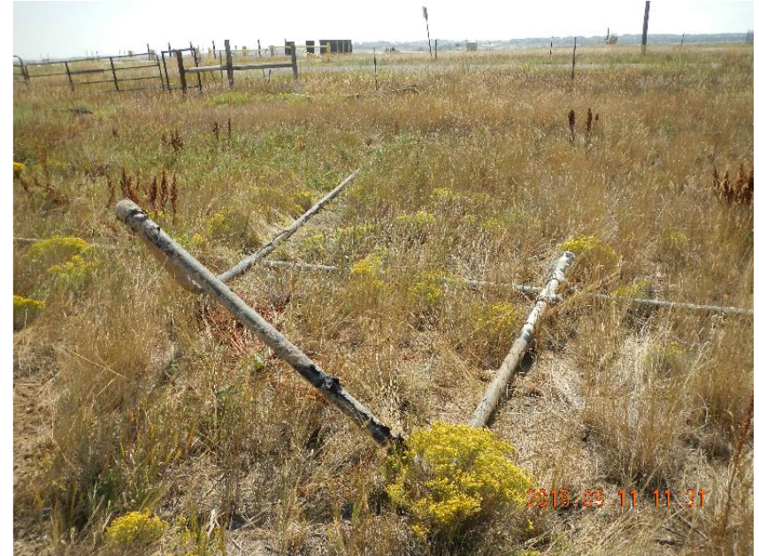
Photo 6: Removed risers and flow lines.
