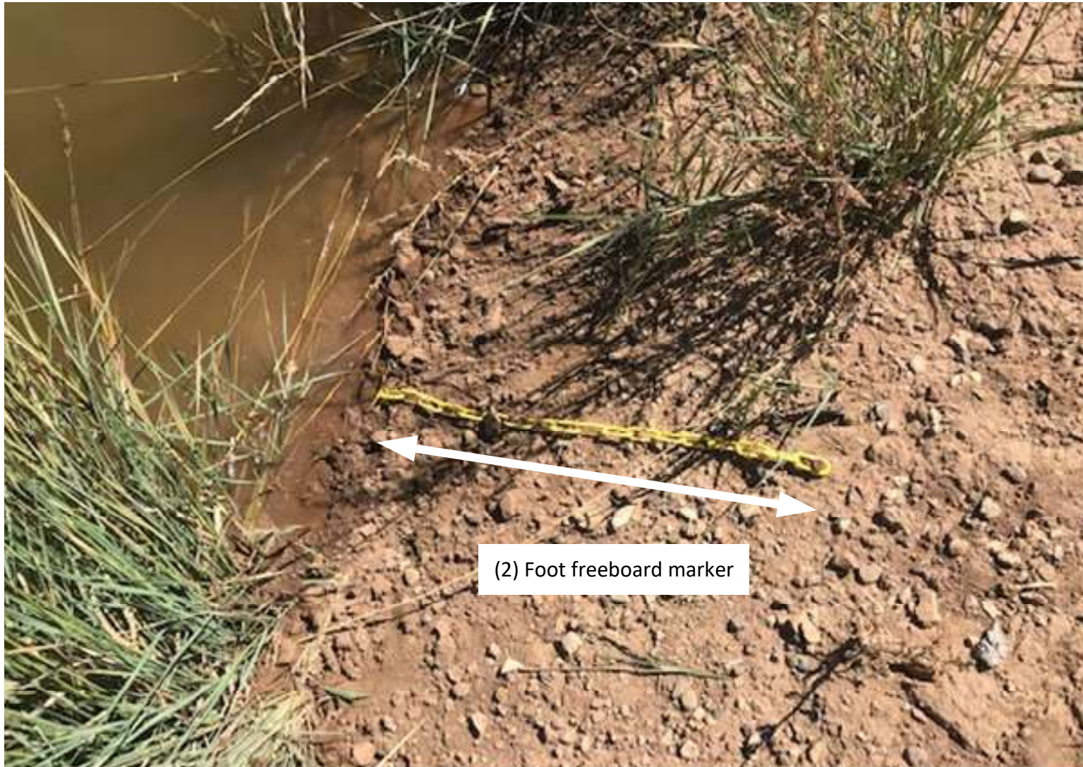
PHOTO 2: Pit level 09/20/19 at 12:27pm. 2 foot freeboard is maintained by disengaging the wellhead. A water truck is in transit to location to remove 20 BBL's of water to provide additional freeboard in the pit.
