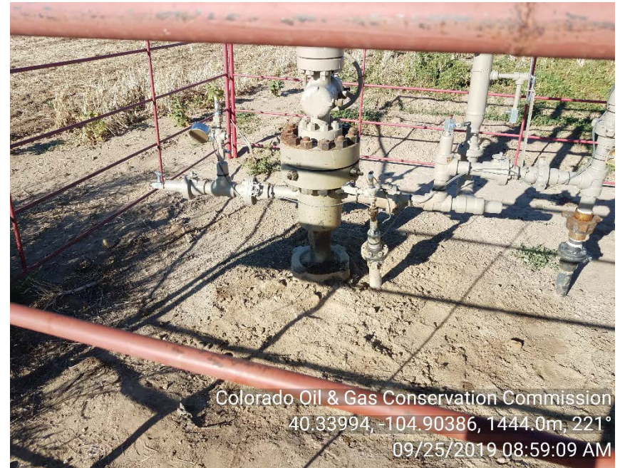
Bradenhead valve and stained soil on 9/25/19
