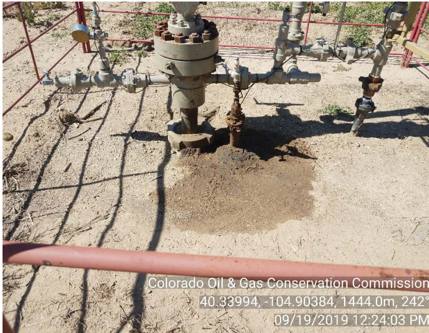
Bradenhead valve and stained soil on 9/19/19
