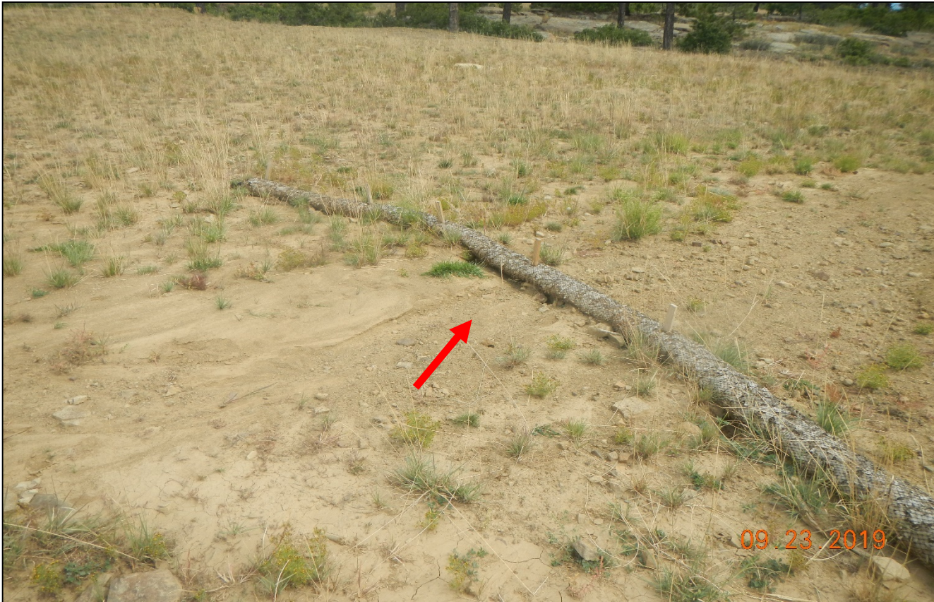
Photo 4. There are sign stormwater is flowing underneath the wattle. Wattles were not properly trenched into the ground. Corrective action was not completed since previous inspection.
