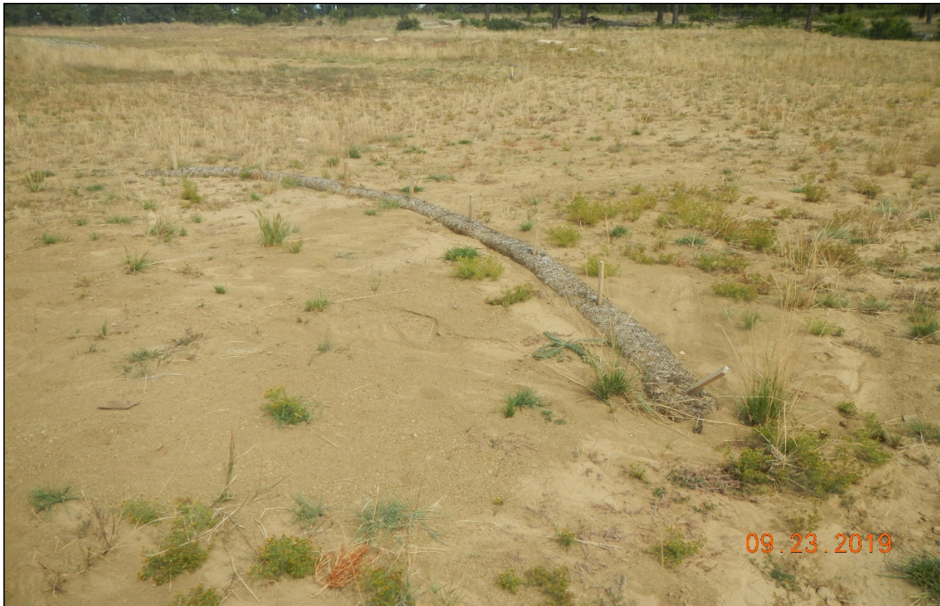
Photo 3. Sediment has filled into the wattles.
