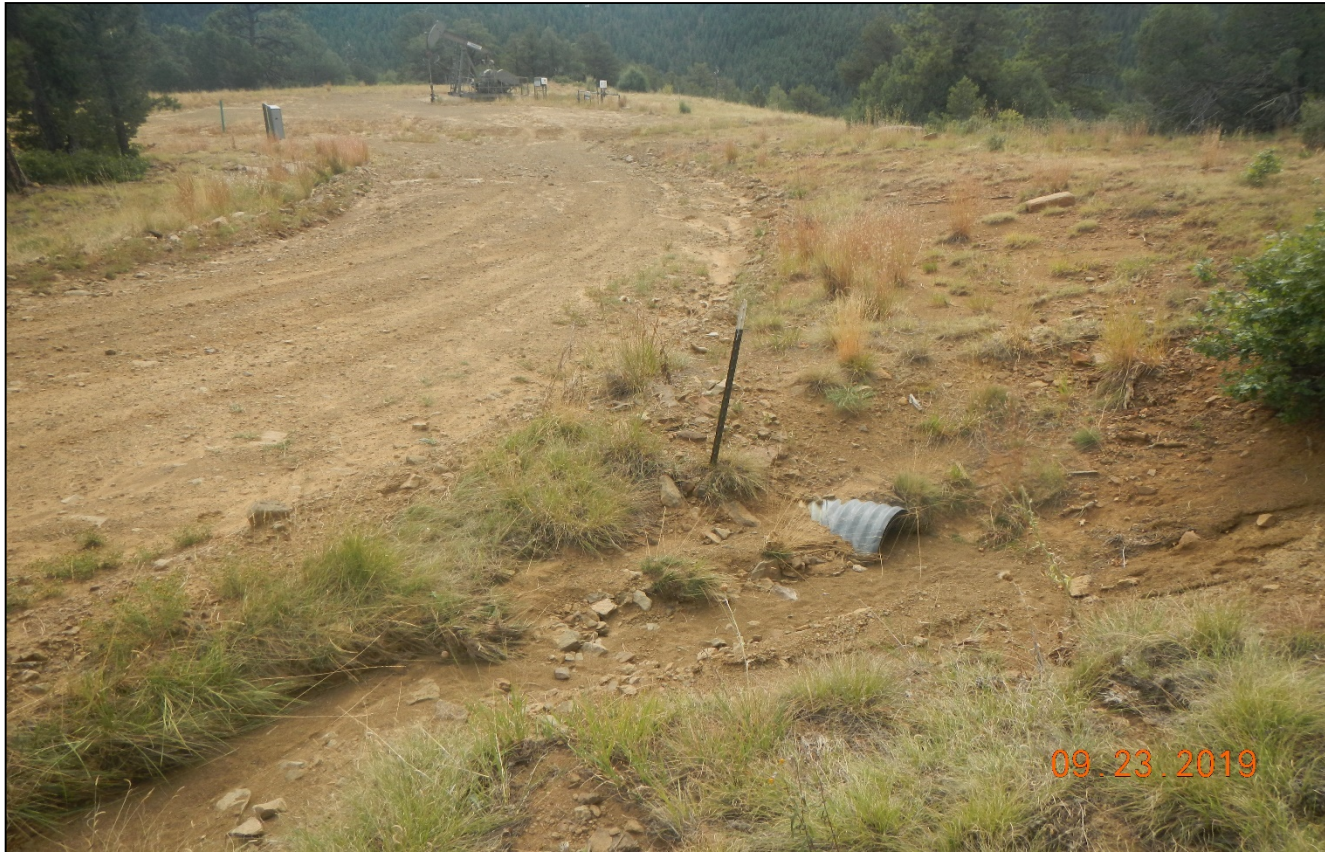
Photo 1. The inlet culvert near the location is partially filled in with sediment.
