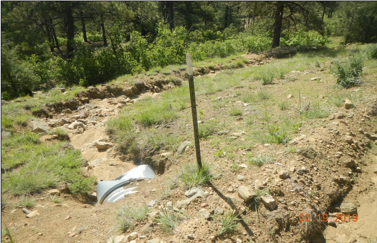
Photo 1. The outlet culvert at the location has no BMP's to prevent erosion. This photo was from previous inspection and was not inspected.
