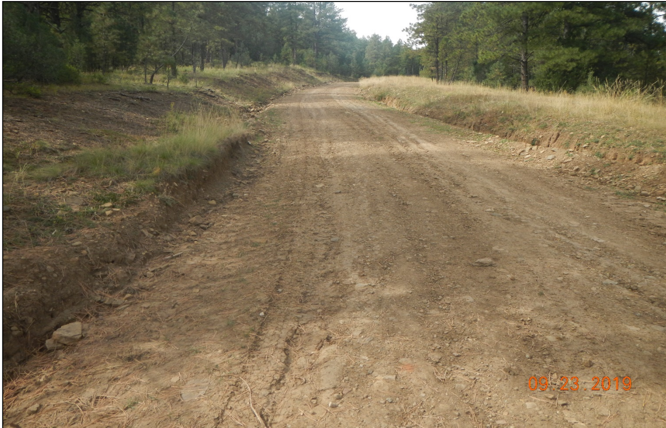
Photo 1. The road has been graded to allow stormwater to drain off the road.
