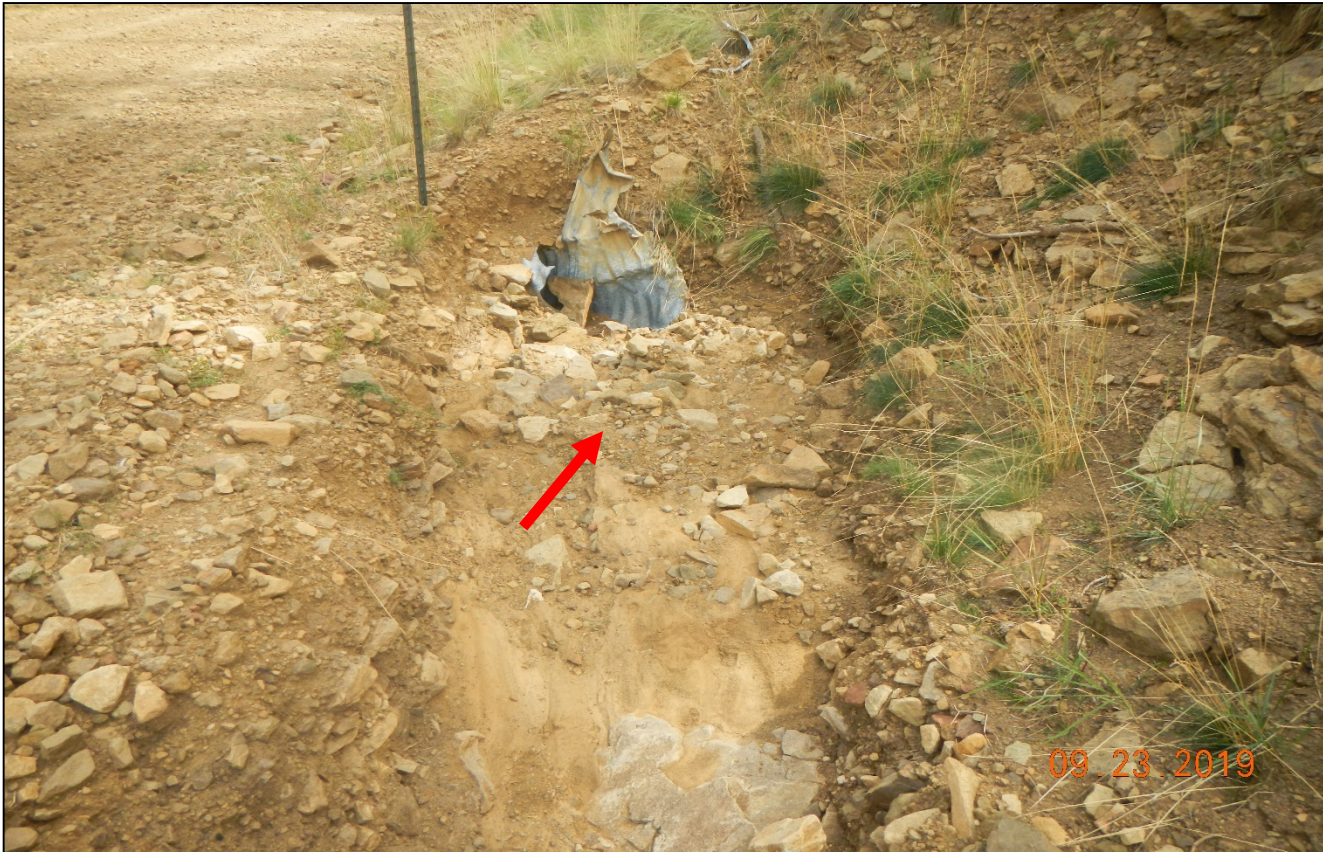
Photo 5. This culvert is partially filled in with sediment and damaged.
