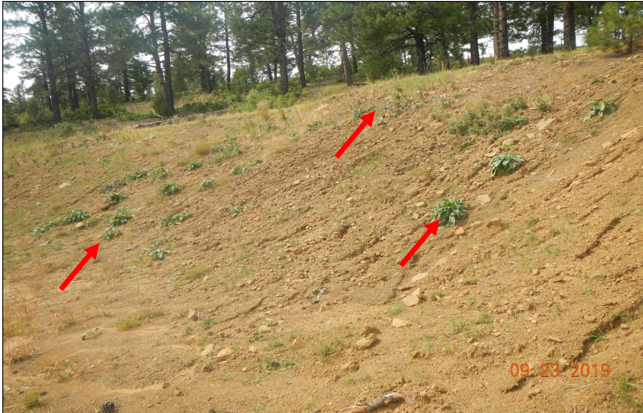
Photo 8. Facing toward the southwest cut slope. Red arrow points to List B noxious weeds. The cut slope is not stabilized. Corrective action was not completed since previous inspection.
