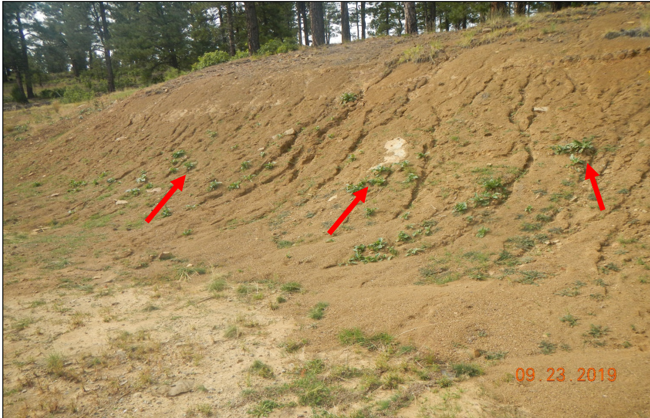
Photo 7. Facing toward the cut slope. Red arrow points to List B noxious weeds. The cut slope is not stabilized. Corrective action was not completed since previous inspection.
