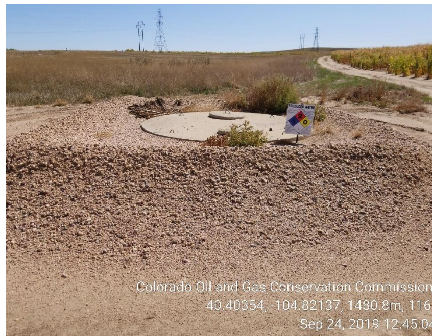
Photo 6: Inadequate berm/Weeds in berm
