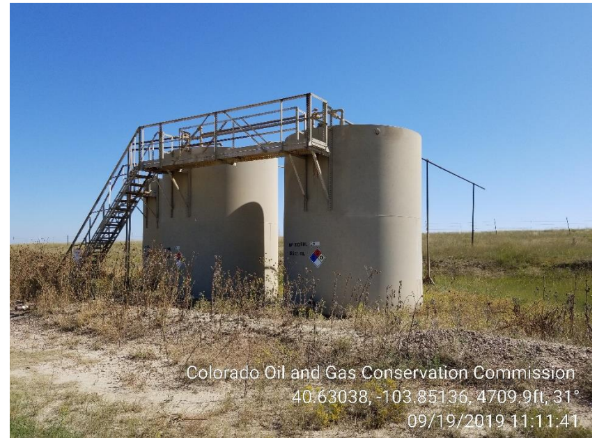
Photo 2 – Tank Battery, weeds actively growing in and out of berm. Tanks are unused equipment
