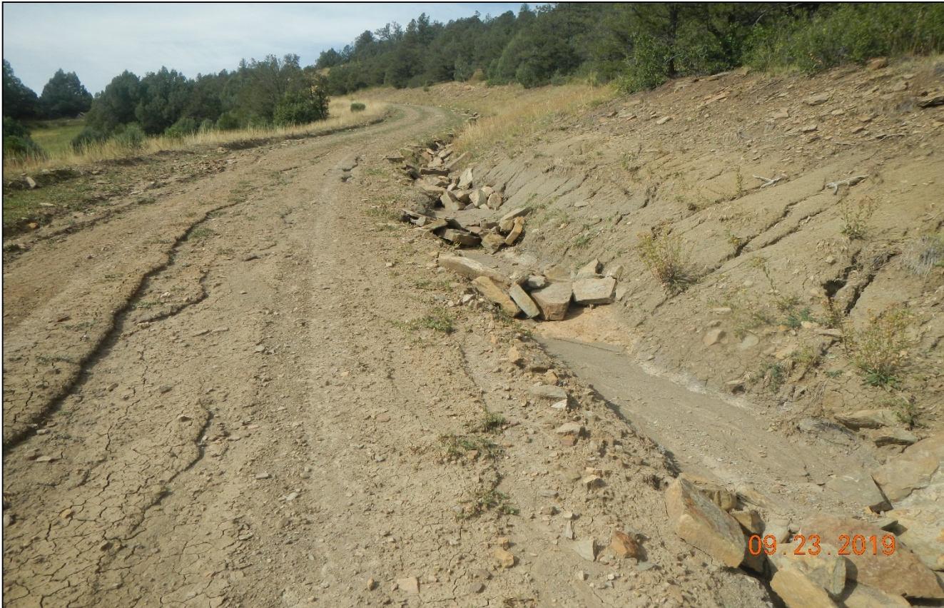
Photo 3. Sediment has filled into the check damns. Erosion is occurring down and along the side of the road. Corrective action was not properly completed since previous inspection.
