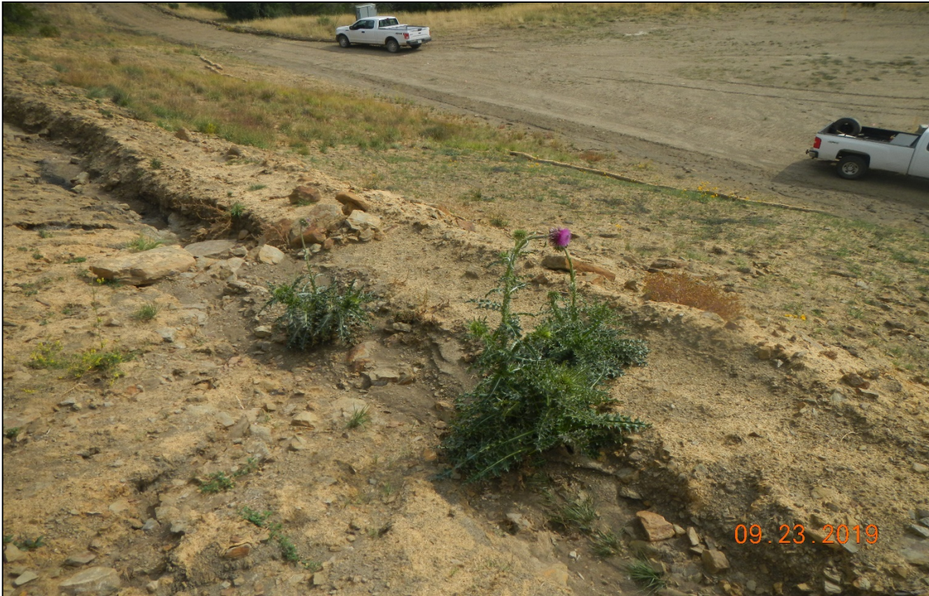
Photo 9. There are noxious weeds (Musk thistle) growing at the top of the cut slope. Corrective action was not completed since previous inspection.
