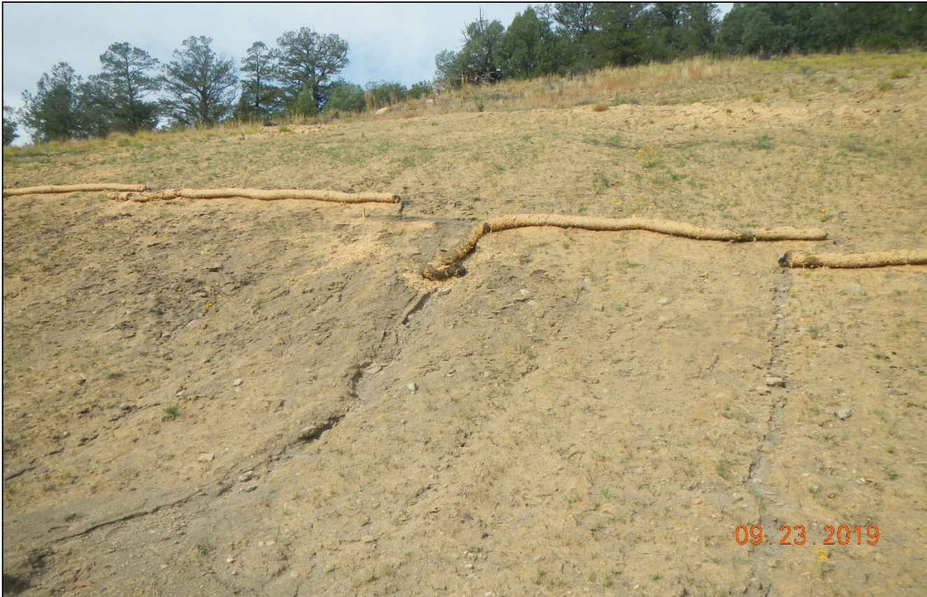
Photo 6. Wattles are displaced along the cut slope.
