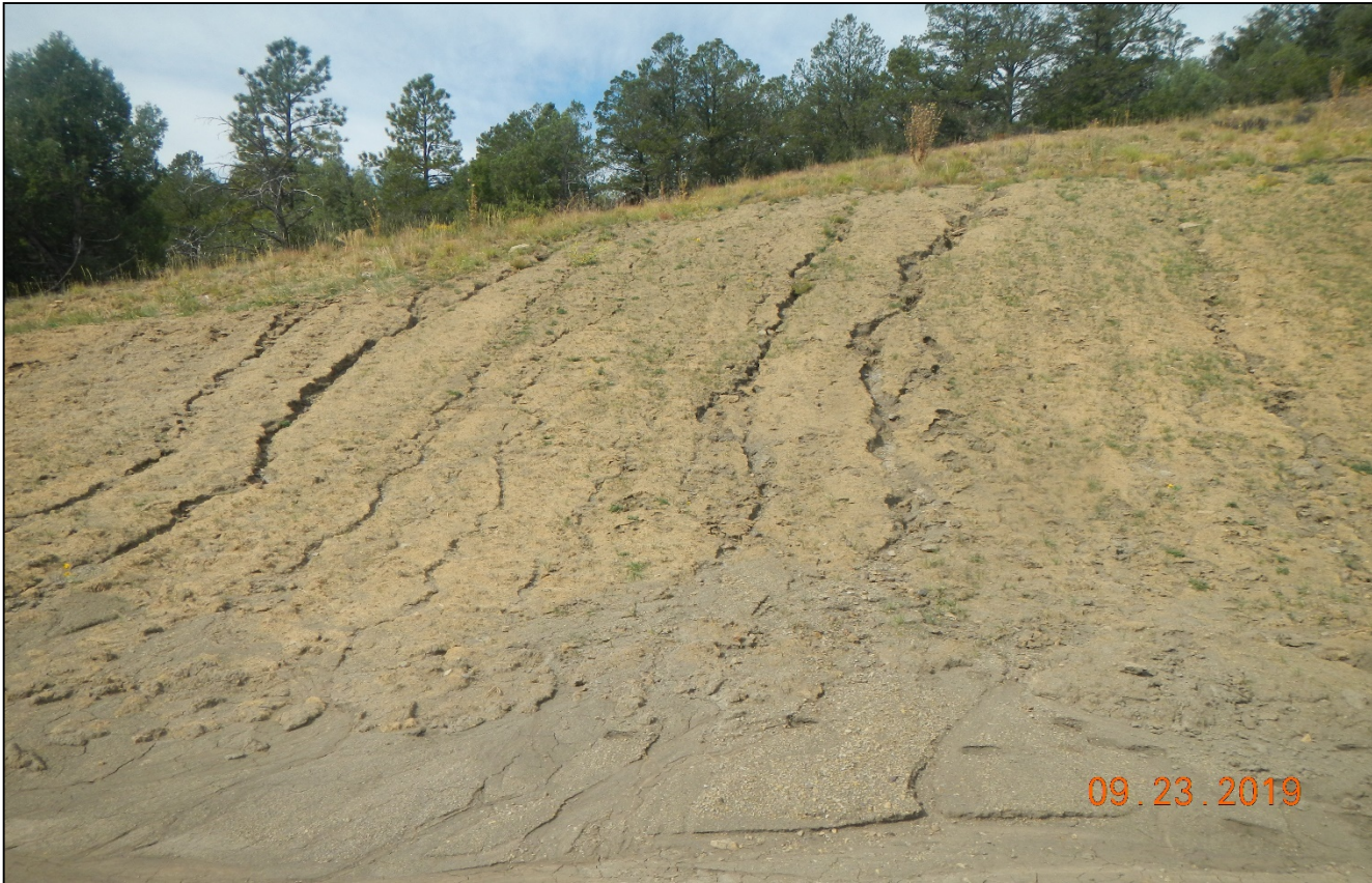
Photo 7. There are erosion channels developing along the cut slope which need to be repaired.
