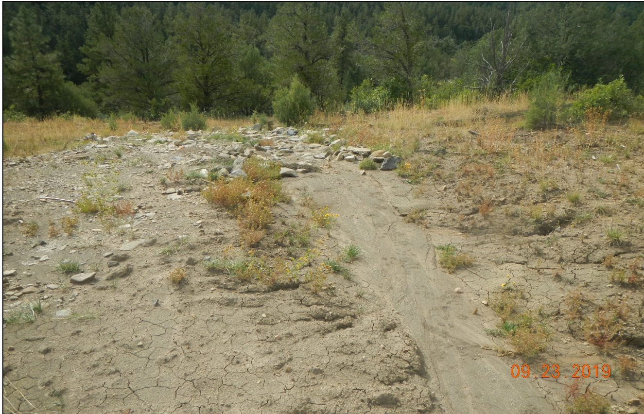
Photo 8. Rock rip/rap was installed at the end of the diversion ditch however, sediment has already filled in the diversion ditch from erosion of the cut slope. Corrective action was not completed since previous inspection.
