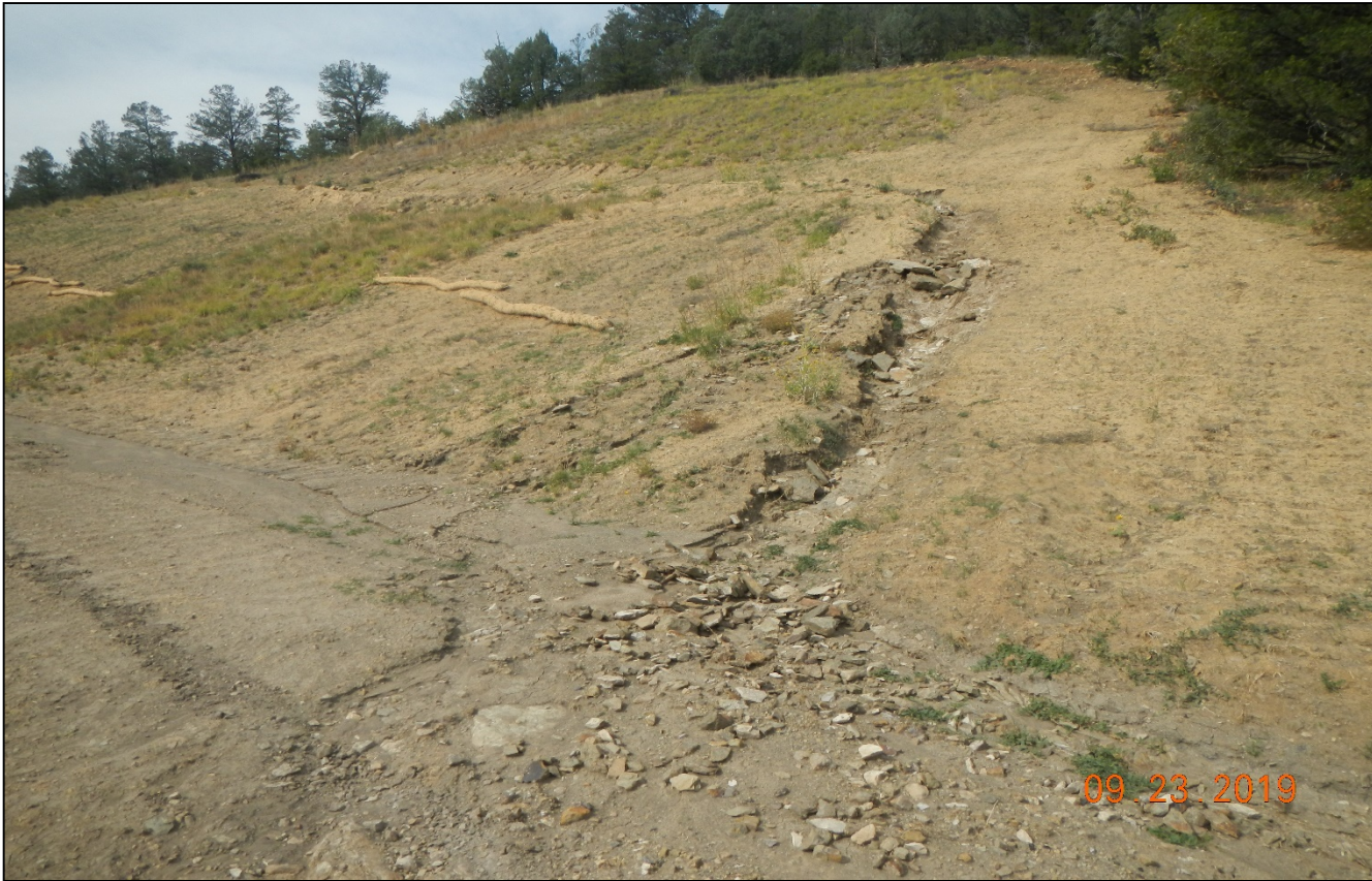
Photo 5. Erosion is occurring down the cut slope from the diversion ditch.
