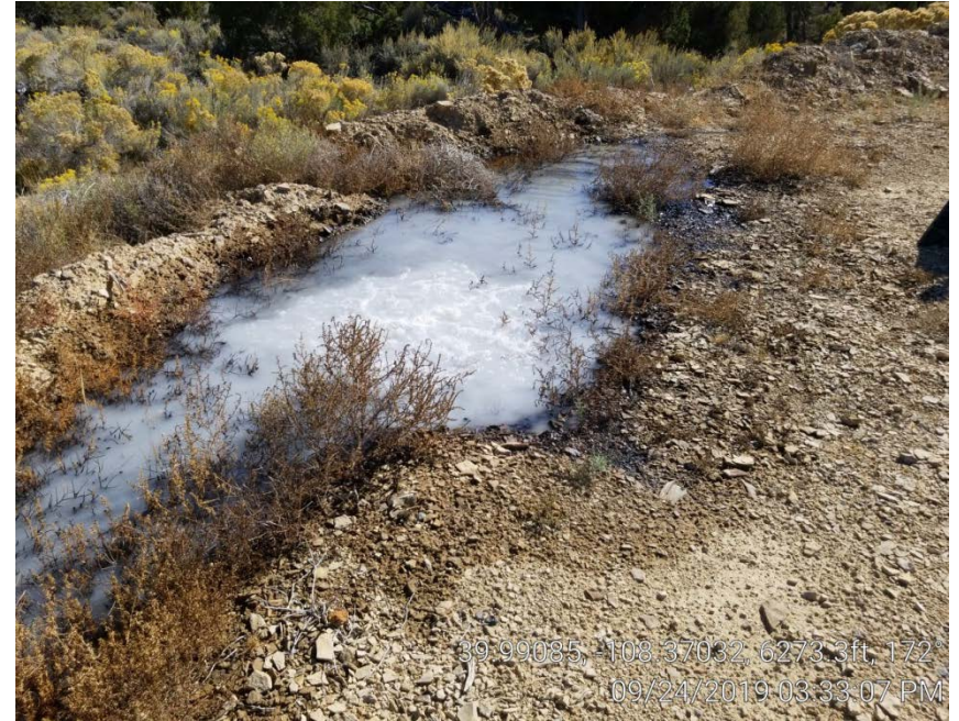
Photo 6. Active leak next to pig station.
