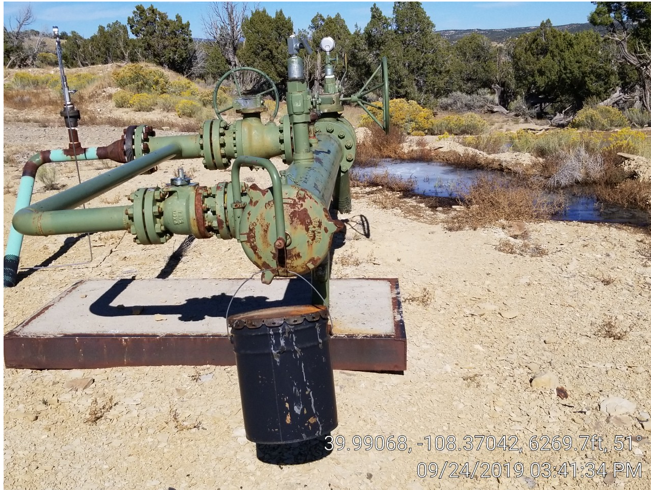
Photo 4. Pig station and active leak.
