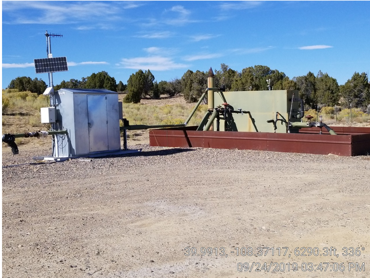
Photo 3. Meter building & separator.
