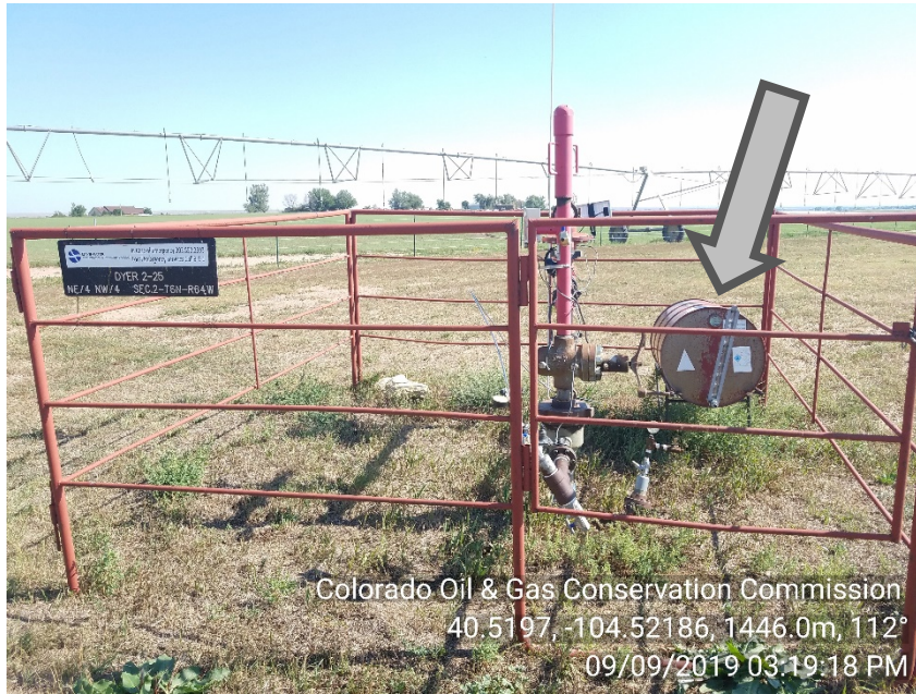
Photo #1 Dyer 2-25 (05-123-28147) Wellsite Shut-In | SI Unused Equipment prior insp.
