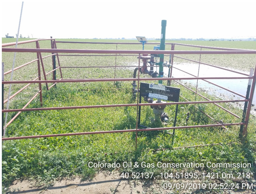
Photo #1 Dyer 2-21 (05-123-28012) Wellsite Shut-In | SI prior insp.
