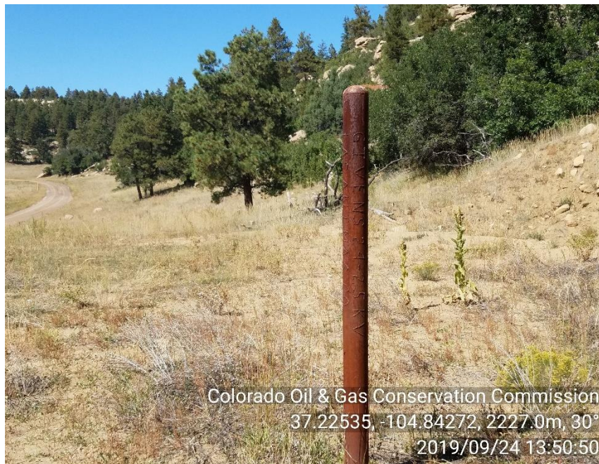
PHOTO 1: WELL IS PA, ABOVE GROUND MARKER
