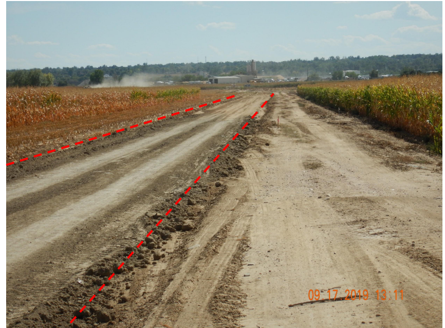
Photo 2. Photo taken from the entrance of the location, facing South. Photo illustrates the Operator has constructed a new access road (red-dashed lines) adjacent to an existing oil and gas access road. Operator indicated that the existing oil and gas access road would be reclaimed. Operator indicated the new access road was a County requirement.
