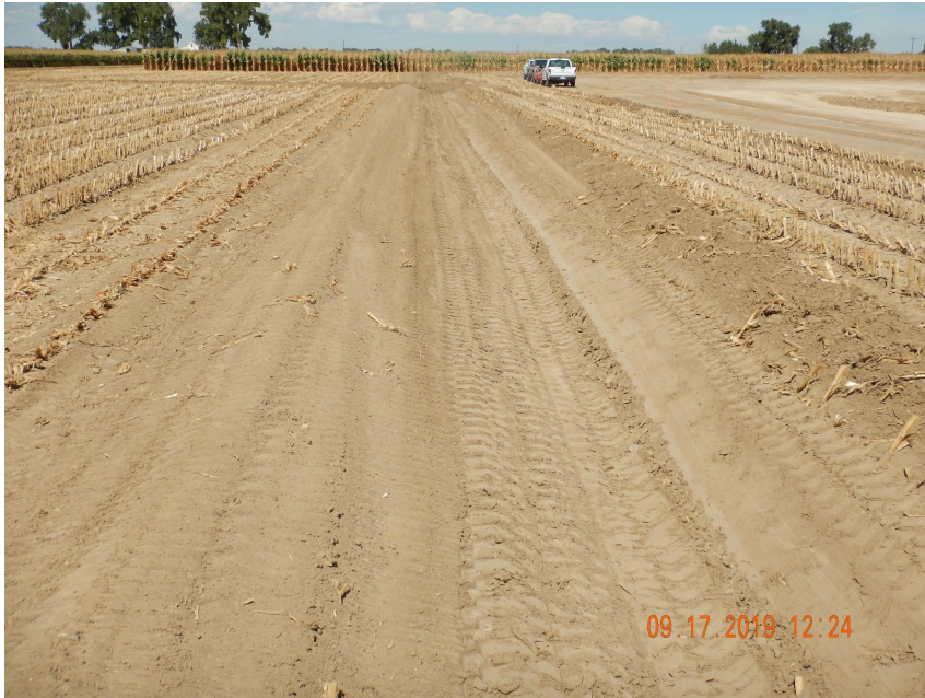
Photo 3. Photo taken from the western well pad location, facing North. Photo illustrates a ditch and berm BMP installed around the perimeter of location. Operator has only constructed the eastern portion of the location.
