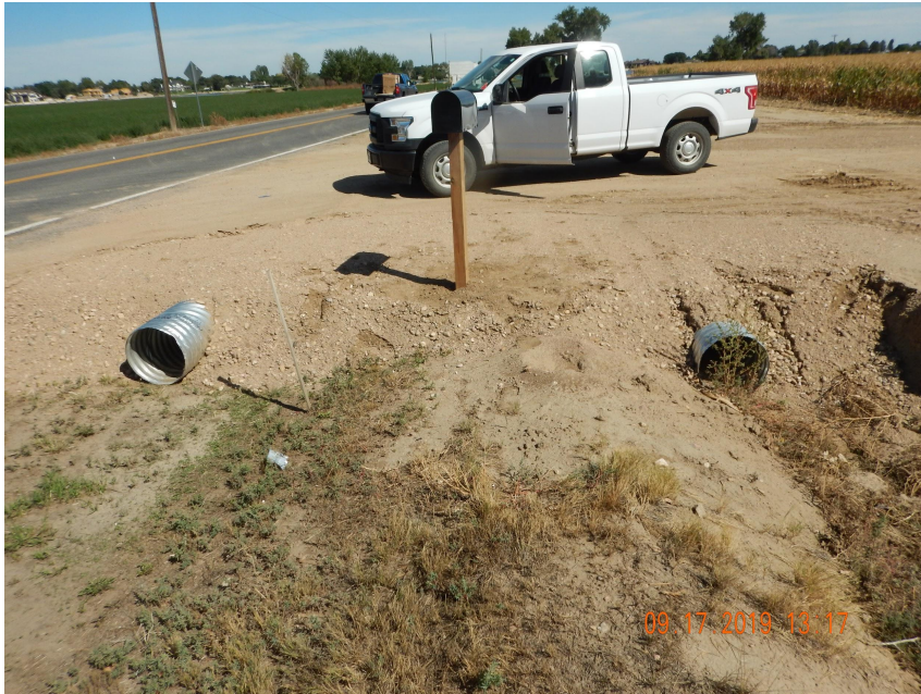
Photo 1. Photo taken from the entrance of the location, facing East. Photo illustrates culverts have been installed. The required permits were inside the mailbox. Operator shall install vehicle tracking device BMPs to ensure compliance with potential sediment discharges from operations, as a new access road has been constructed.
