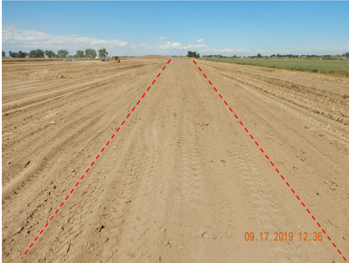
Photo 7. Photo taken from the eastern well pad location, facing North. Photo illustrates a topsoil stockpile (red-dashed lines) stored along the eastern perimeter.
